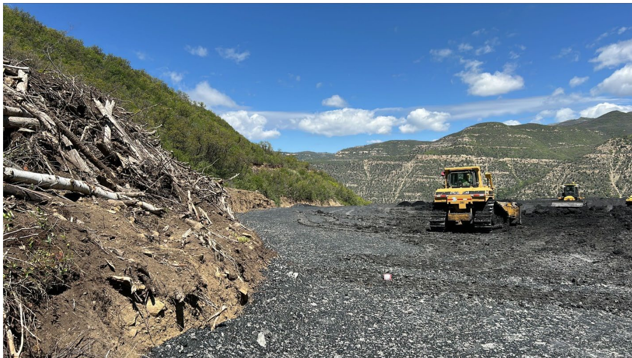
Figure 13: Compaction of processing waste in progress
