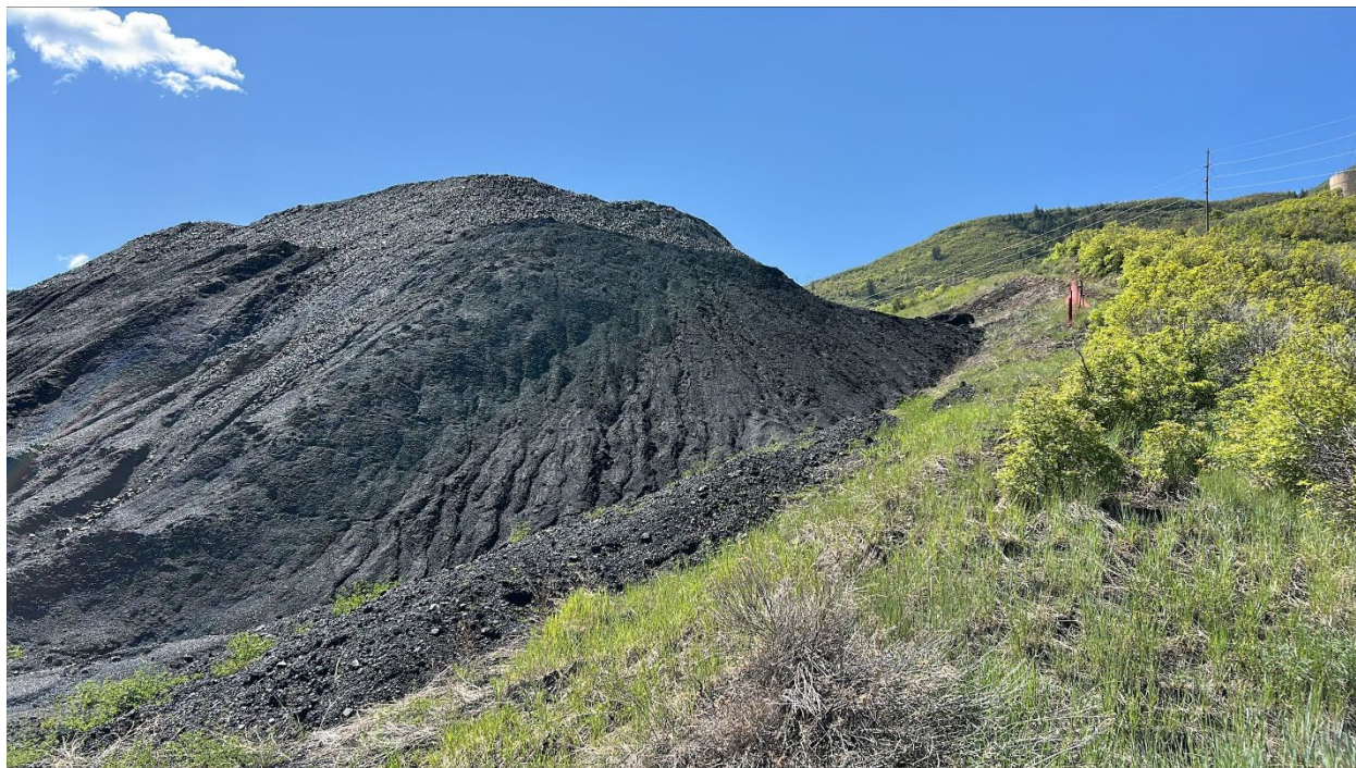
Figure 4: Western end of Run-of-Mine coal stockpile pad; material retained within pad footprint.
