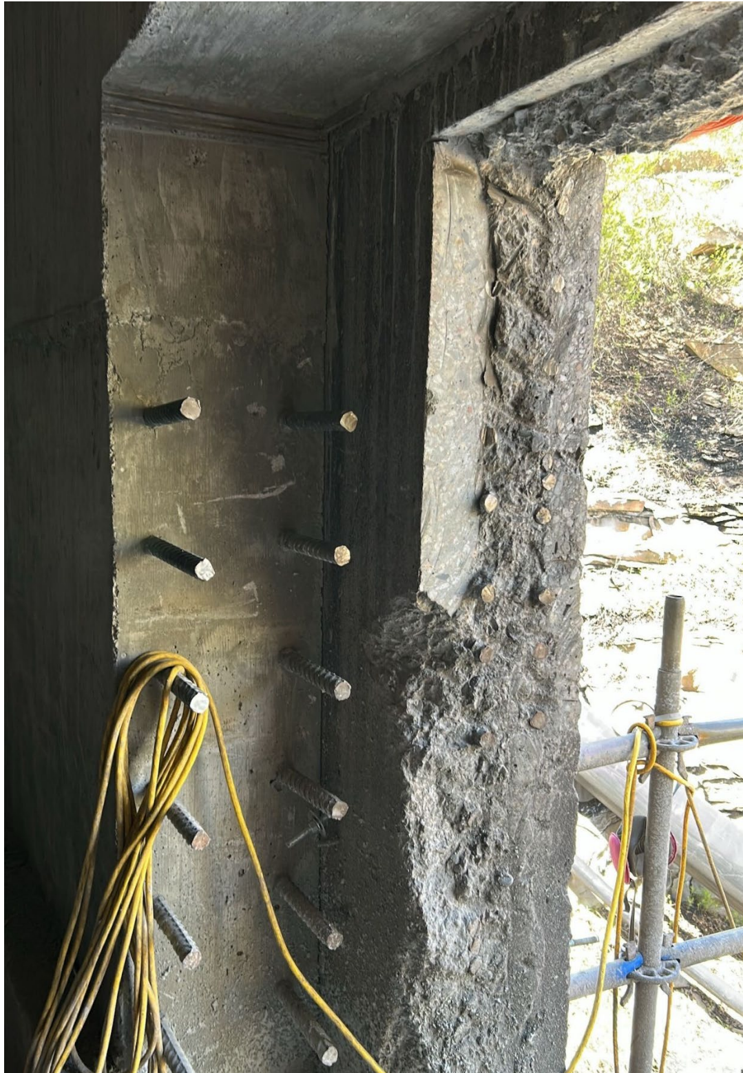
Figure 8: Wall of silo, showing original concrete(R) and new lining(L)
