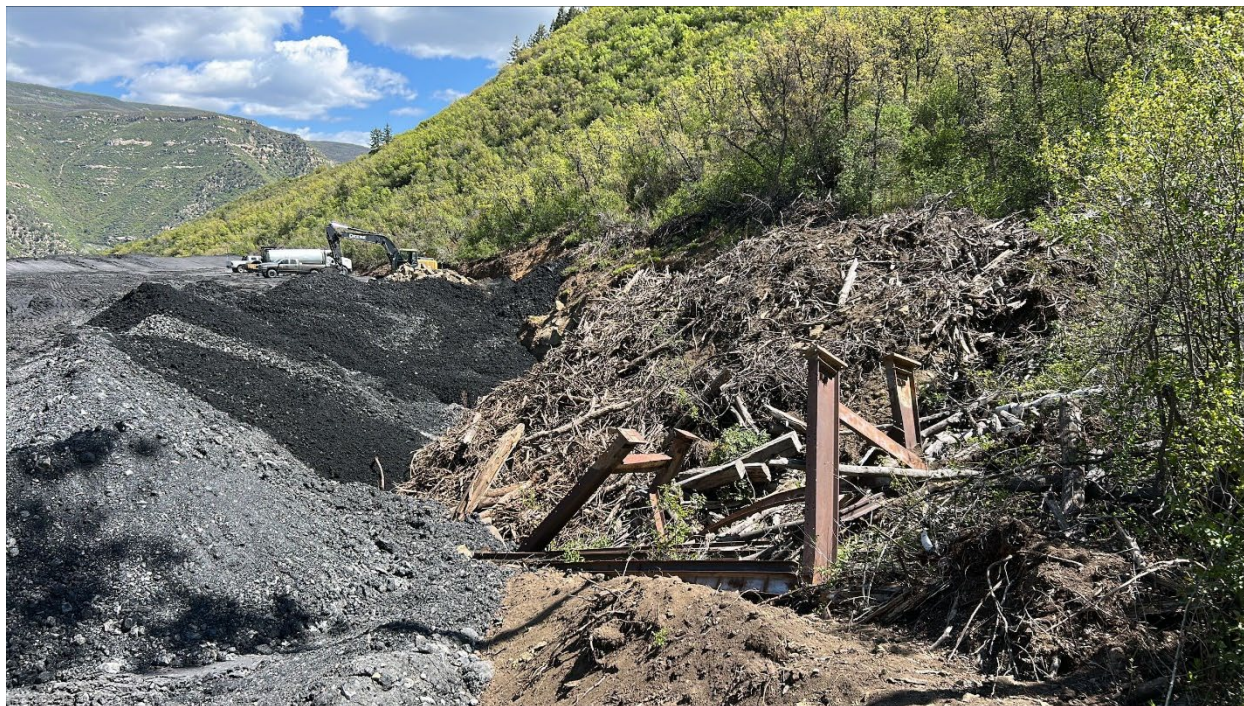
Figure 12: Grubbed vegetation and scrap metal at southeast edge of RPEE must be removed before refuse can be placed
