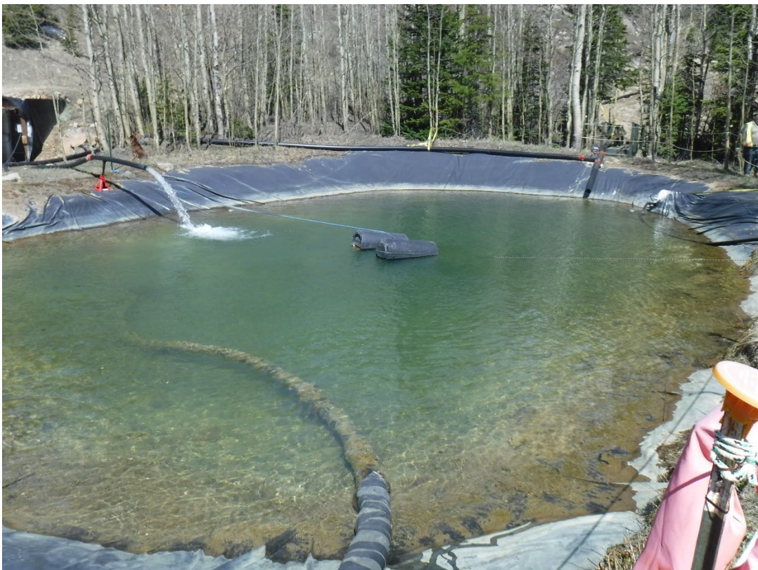
Photo 4: Pond 1 with the Joliet Raise inflow and Idaho Tunnel effluent being direct to the Raise
