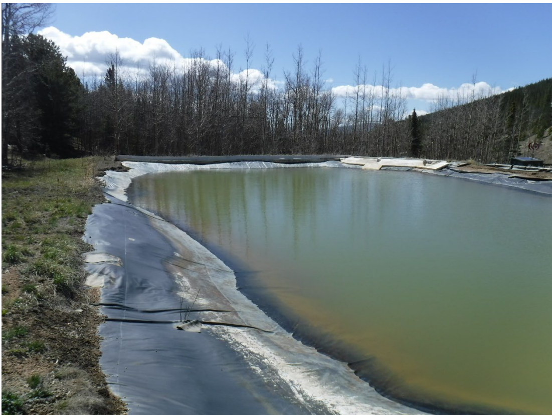
Photo 6: Pond 2 looking south
