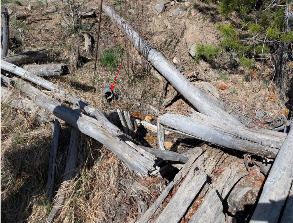
Photo 9: Looking at the overflow pipe for the seepage collection system below the engineered spillway.
