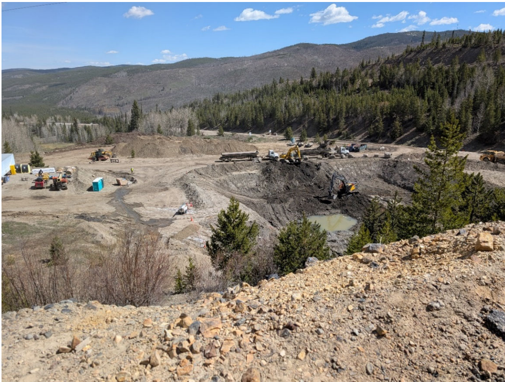
Photo 17: Standing on a ledge along the north side of the Mill looking down at the excavation work for the foundation of the future Water Treatment Plant.
