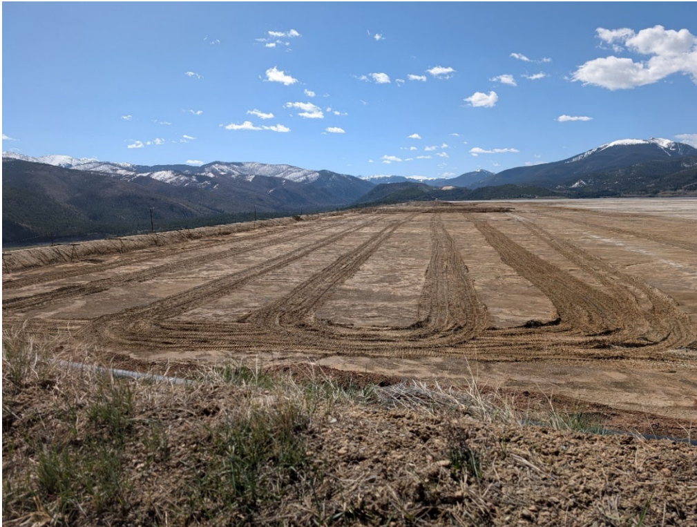
Photo 16: Looking south across the Tailings Storage Facility from the north end of 1-Dam. The tire tracks are associated with the use of Coherex for dust suppression which was recently spread across the tailings deposition area.
