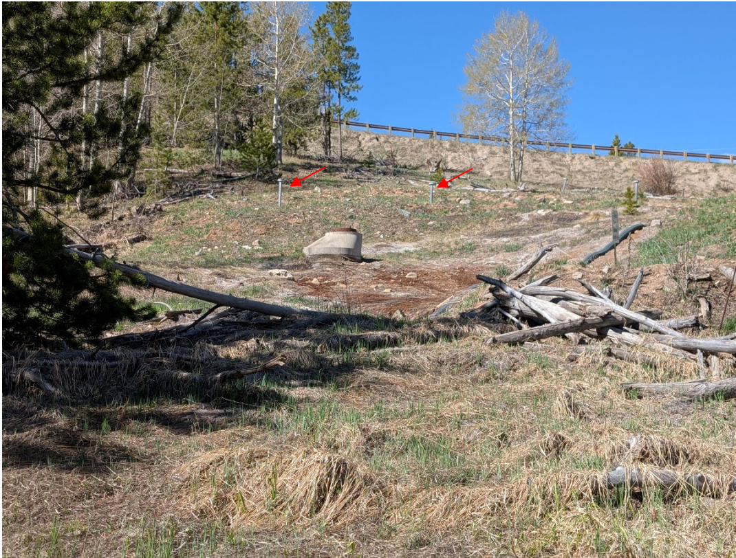
Photo 5: Looking up at the seepwater collection area below 3-Dam. French drains (red arrows) collect seep water and funnel it to the collection system vaults to the pipelines.
