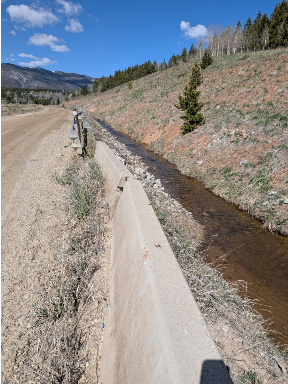
Photo 15: Looking west at the ultimate canal on the north end of the TSF where a pipeline is proposed to be installed.
