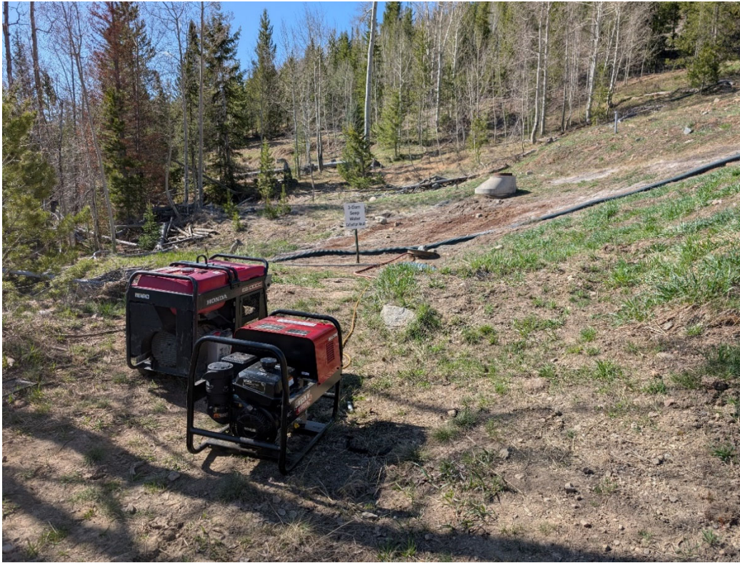
Photo 7: Generators observed in the area of the containment area.
