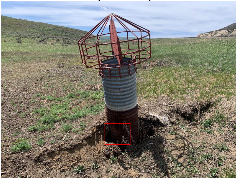
Photo 2- Pond T primary spillway needs to be maintained. See close-up of red square in Photo 3
