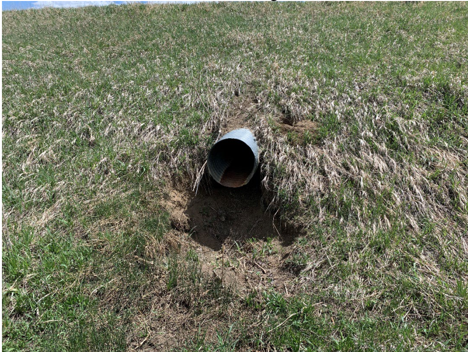
Photo 4- Pond T primary spillway outlet pipe
