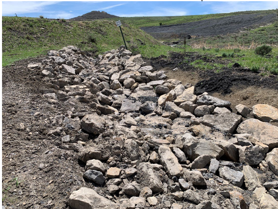
Photo 8- Rock lined ditch from the BOB to Pond B sump
