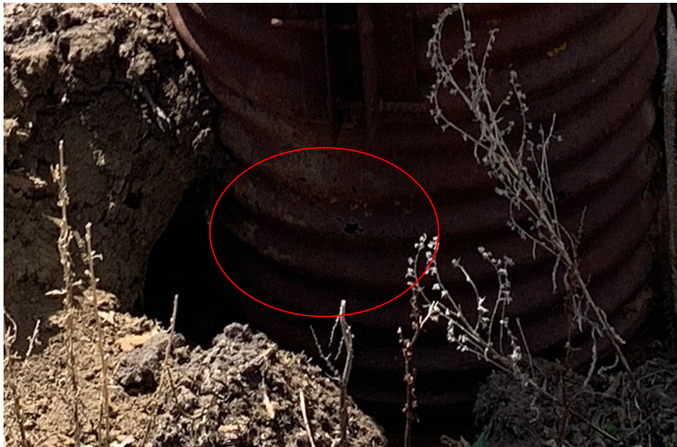
Photo 3- Holes rusted through culvert metal.
