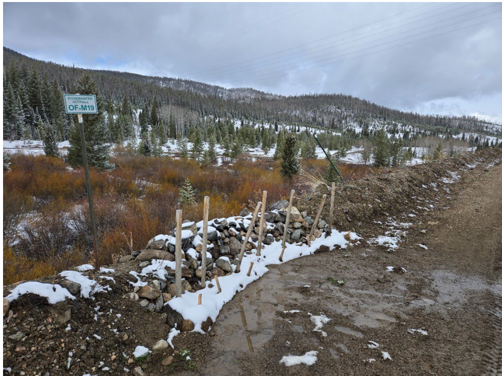
OF-M19 (Photo 15) - The BMPs of this outfall location consist of wattles in front of a rock check dam leading to a rip-rap outfall. This outfall location appears to be in good condition.
