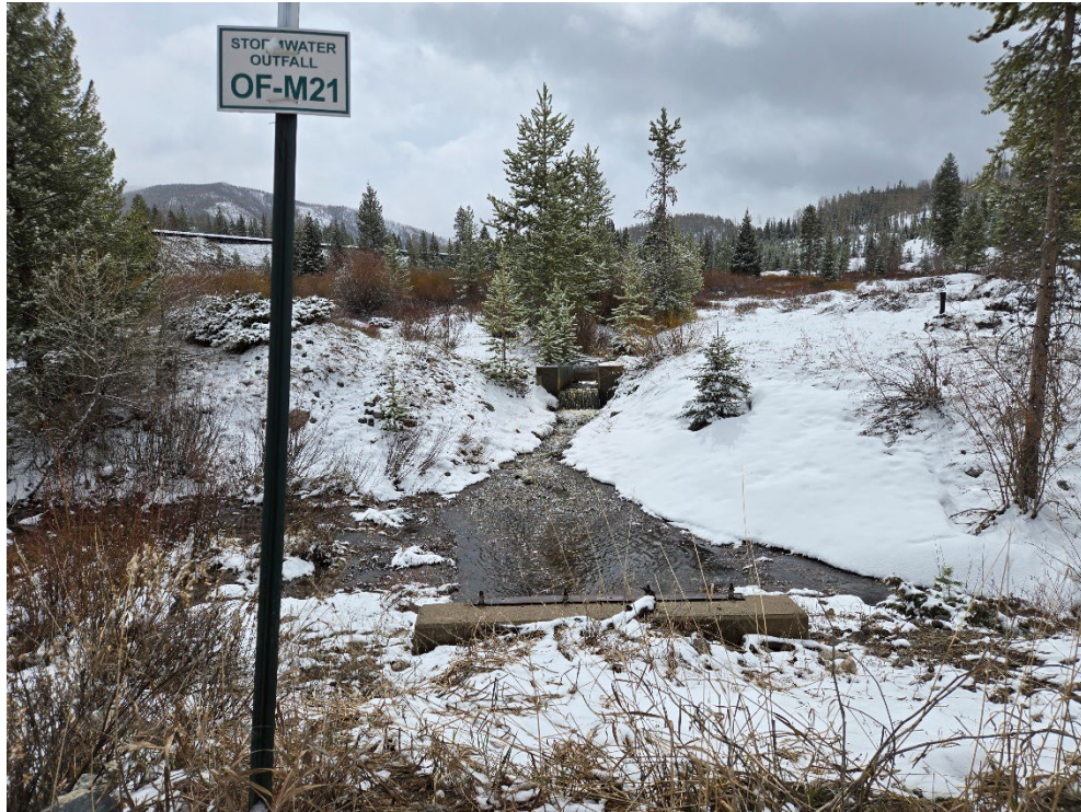
OF-M21 (Photo 14) - The BMPs of this outfall location consist of wattles in front of a rock check dam leading to a rip-rap outfall. This outfall location appears to be in good condition. This outfall is located west of what is depicted on the SWMP maps.
