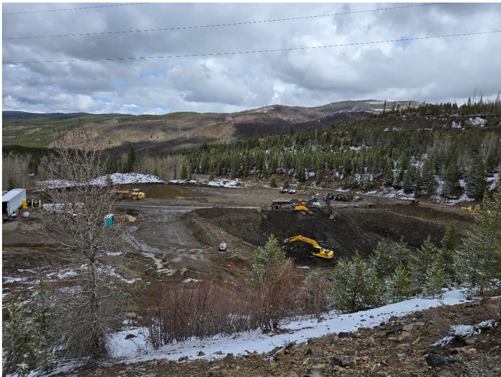
Photo 24: Current progress made on the construction of the new water treatment plant approved through TR35. During the inspection, equipment was being used to conduct some pre-building clean up and excavating debris. The Operator stated that soil testing had recently been conducted to determine whether there were any materials previously buried in this area.
