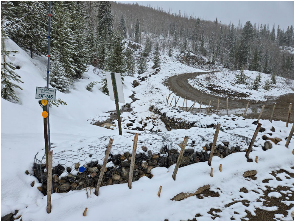
OF-M05 (Photo 9) - The BMPs of this outfall location consist of wattles in front of a rock check dam. Stormwater that goes through this structure converges with clean water coming from the south. Water then
