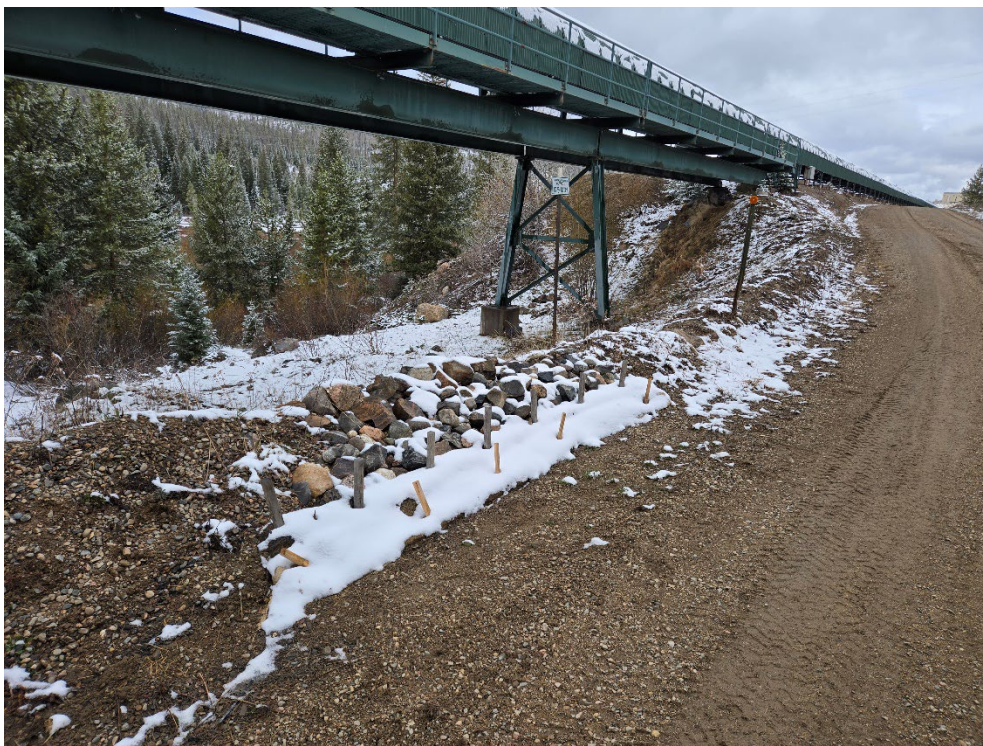
OF-M31 (Photo 17) - The BMPs of this outfall location consist of wattles in front of a rock check dam leading to a rip-rap outfall. No water was moving through this structure during the inspection. The Operator stated that this outfall does not experience a lot of flow. This outfall location appears to be in good condition.
