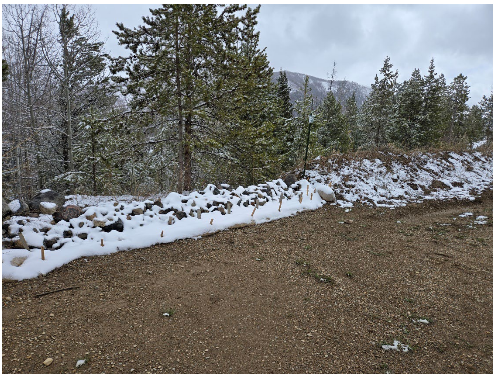
OF-M30 (Photo 19) - The BMPs of this outfall location consist of wattles in front of a rock check dam leading to a rip-rap outfall. This outfall collects drainage from the northwest lay down area areas and the southeast side of the road. However, the area did not hold water or excess sediment at the time of the inspection. This outfall
