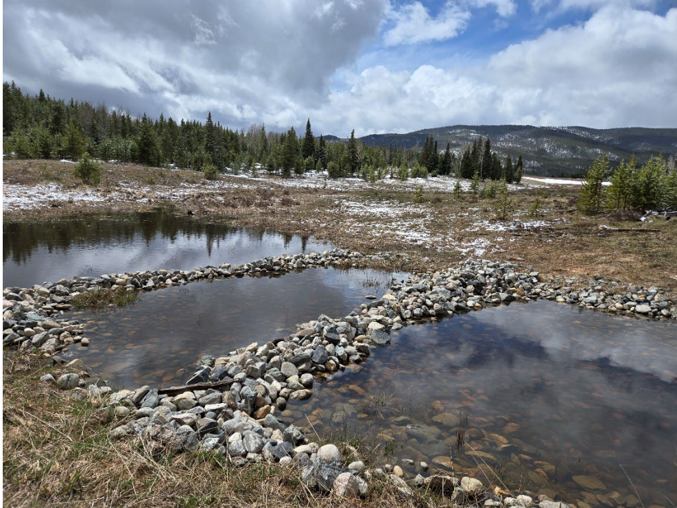
(Photo 23) - A series of check dams lead to OF-M29 and discharge into the pond seen in Photo 22 through a culvert that goes under the road.
