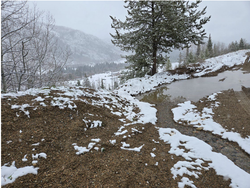
OF-M07 (Photo 6) - The BMPs of this outfall location consist of wattles in front of a rock check dam leading to a rip-rap outfall. The Division observed water moving through this structure during the inspection. The wattles were covered in snow and it was difficult to assess their condition, but this outfall location appeared to be working well.
