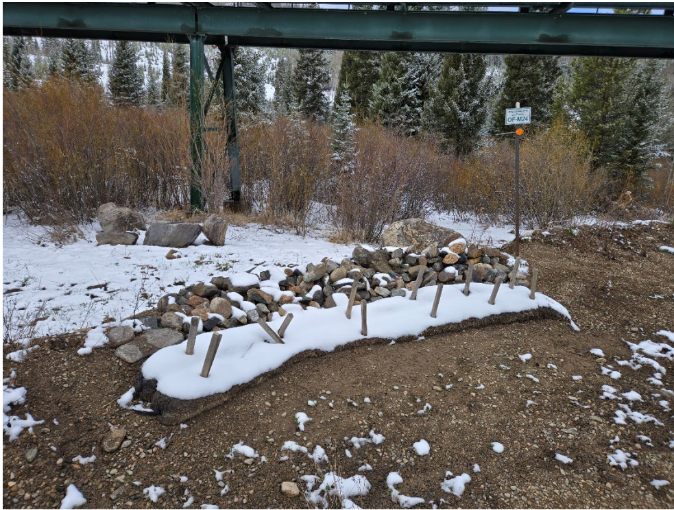
OF-M24 (Photo 18) - The BMPs of this outfall location consist of wattles in front of a rock check dam leading to a rip-rap outfall. This outfall collects drainage from the north side of the road, but it does not appear that it had experienced much runoff recently. This outfall location appears to be in good condition.
