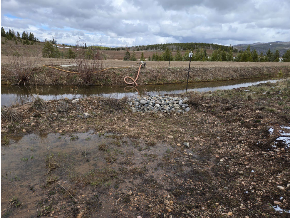
OF-M32 (Photo 21) - The BMPs of this outfall location consist of riprap, and a shallow basin. The basin held a little bit of water at the time of the inspection, and no water was discharging at the outfall.
