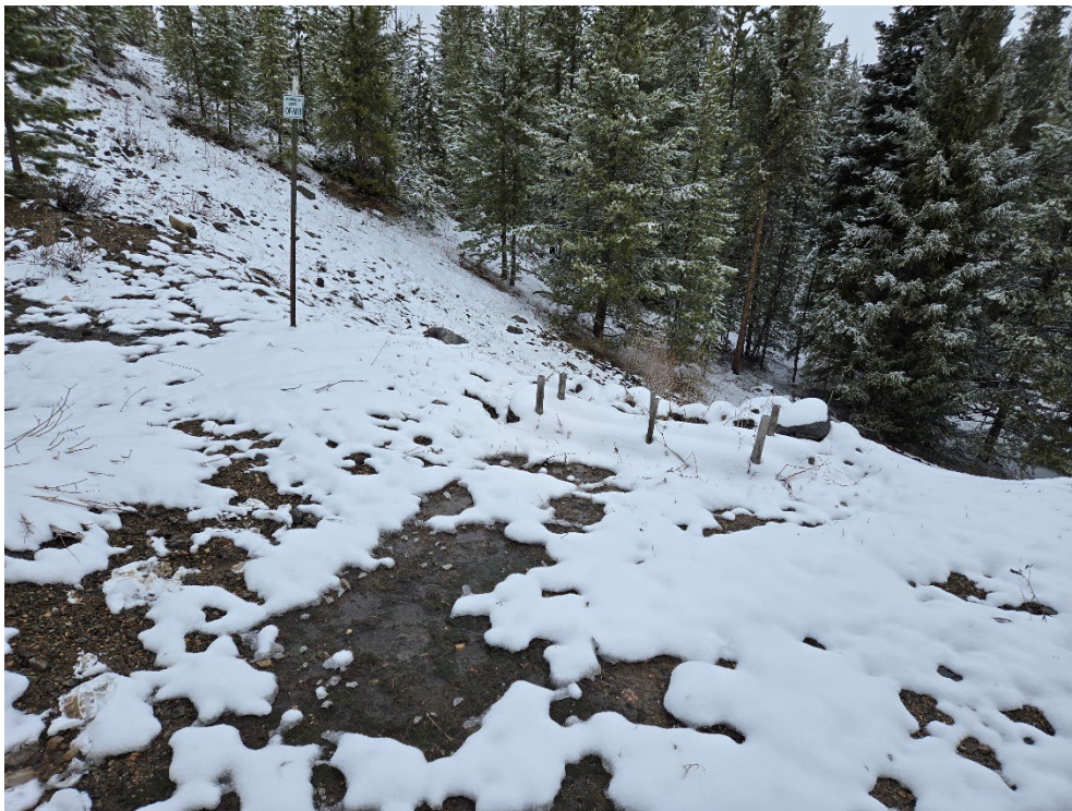
OF-M18 (Photo 13) - The BMP at this outfall location consisted of riprap, which was covered with snow at the time of inspection. The Operator stated that this outfall does not experience much flow.
