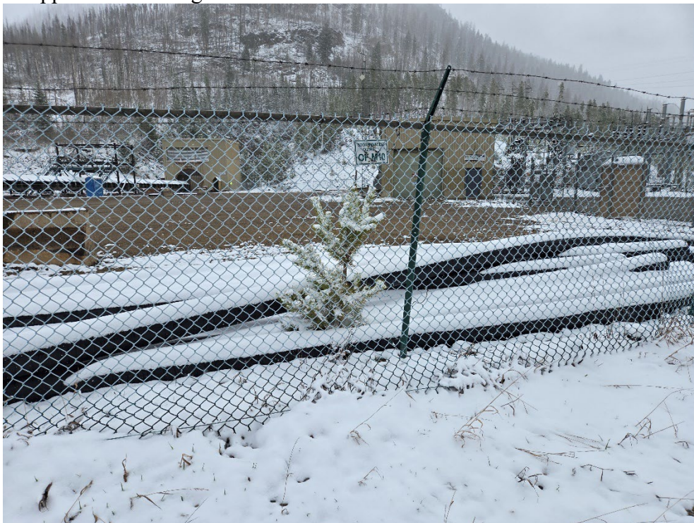
OF-M10 (Photo 5) – This is a low spot near the lay down yard where water may accumulate. However, this outfall does not experience a lot of flow. The BMPs of this outfall location consist of riprap, which was covered with snow at the time of inspection.
