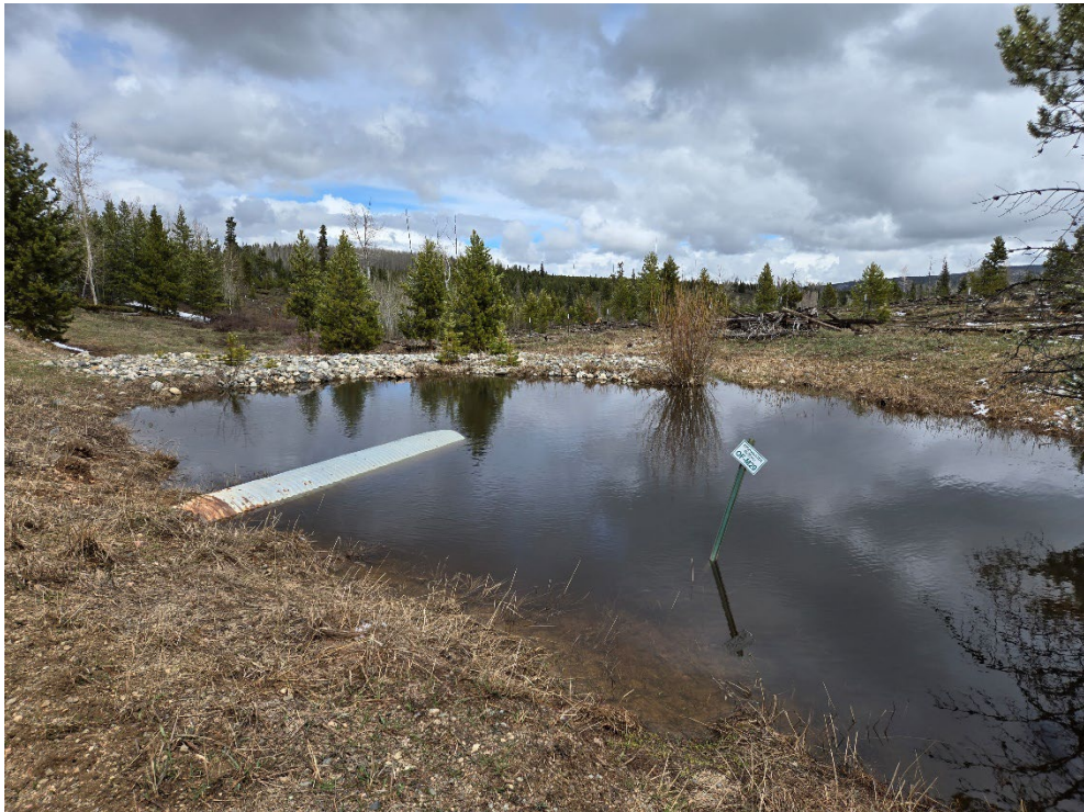
OF-M29 (Photo 22) – The BMPs at this location consisted of a settling pond and a rip-rapped bank. The pond held water at the time of the inspection. This outfall appeared to be in good condition.
