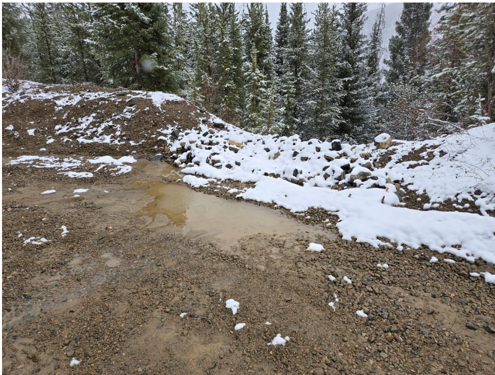
OF-M12 (Photo 7) - The BMPs of this outfall location consist of wattles in front of a rock check dam leading to a rip-rap outfall. The Division observed water moving through this structure during the inspection. This outfall location appears to be in good condition.
