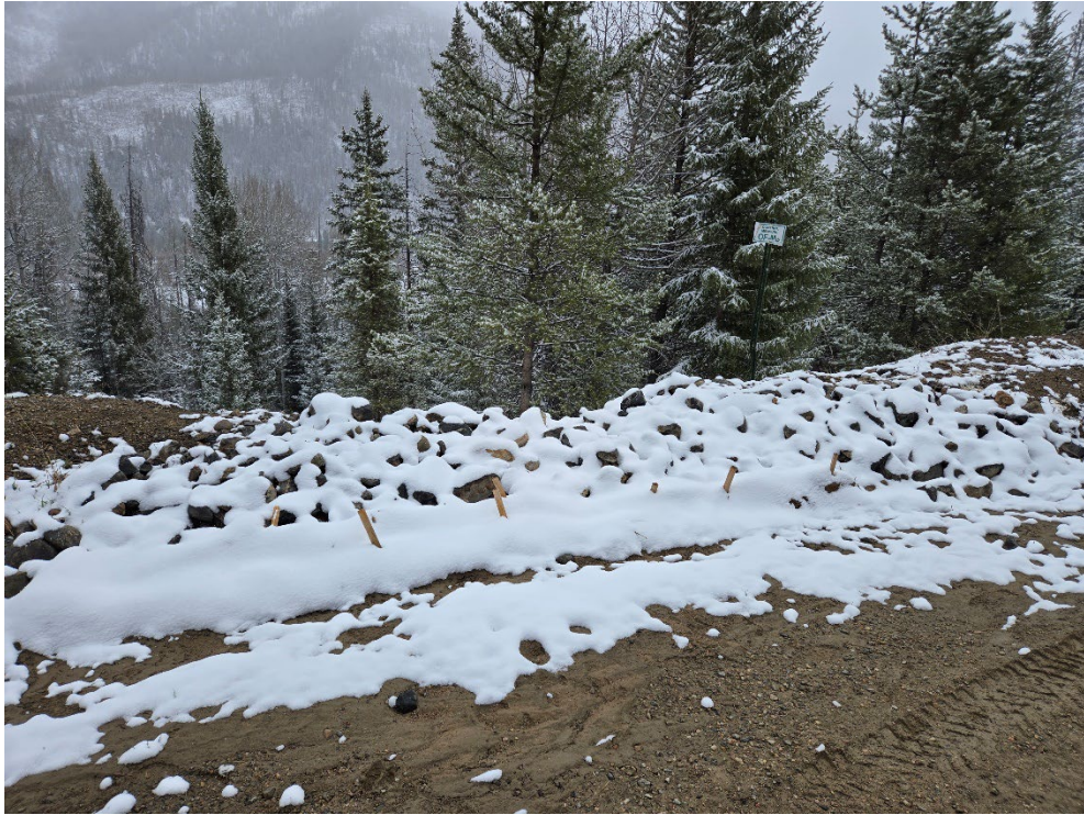
OF-M06 (Photo 8) - The BMPs of this outfall location consist of wattles in front of a rock check dam leading to a rip-rap outfall. No water was observed moving through this structure during the inspection. This outfall location appears to be in good condition. The sign was damaged, but the Operator has already ordered new signs.
