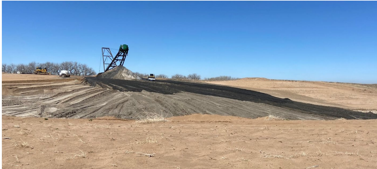
Figure 4.2: Stockpile Development Constructed from Cyclone Underflow
