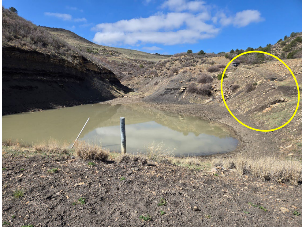
Photo 3: Looking south at Pond 08. Circled is the erosion on the west banks.
