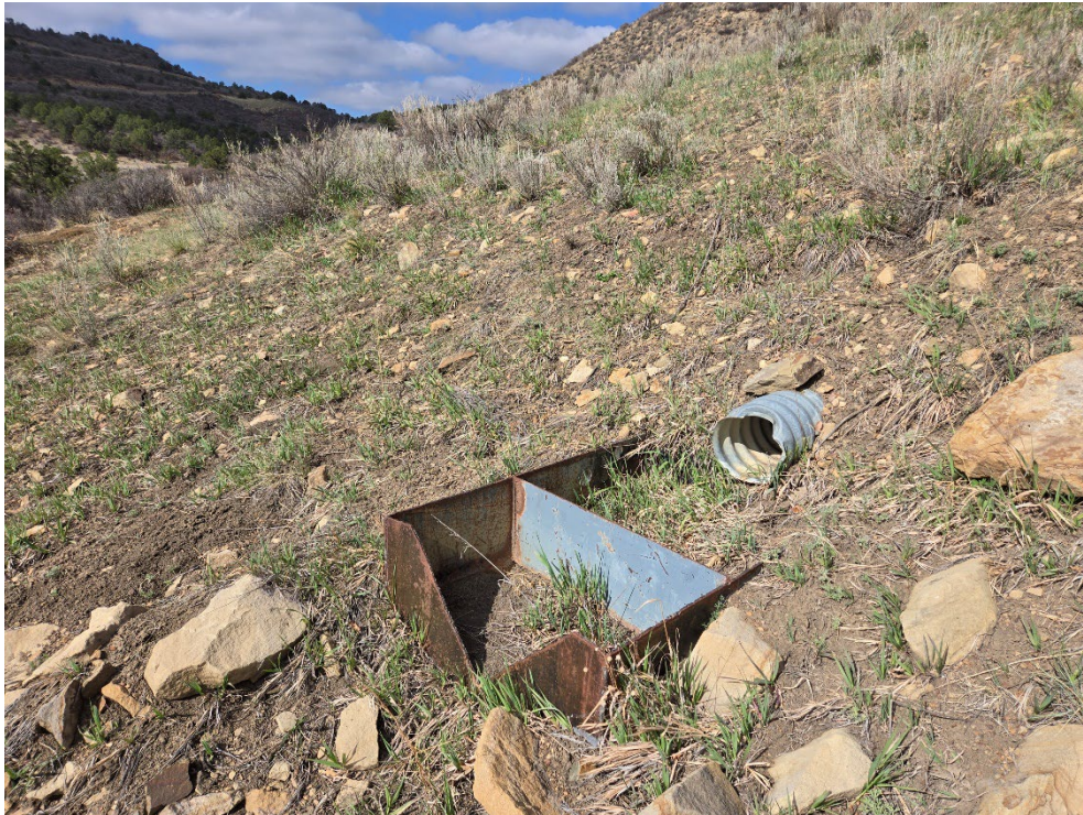
Photo 11: Looking west at the sediment accumulated in the flume for Pond 006a.
