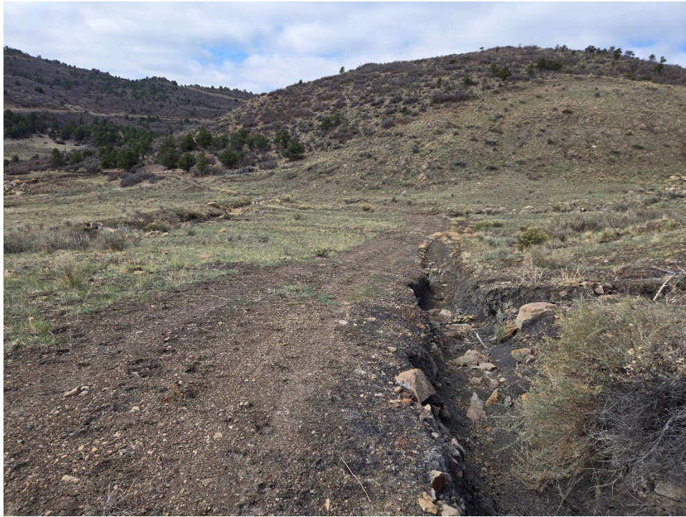
Photo 8: Erosion cutting into the north side of the road leading down to Pond 006a.
