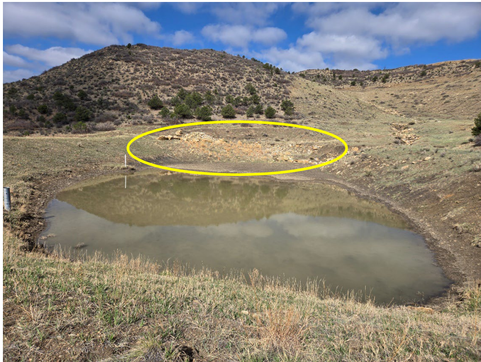
Photo 1: Pond 006a looking west. The western erosion appears to have volunteer vegetation cover that is aiding in stabilization (yellow circle).
