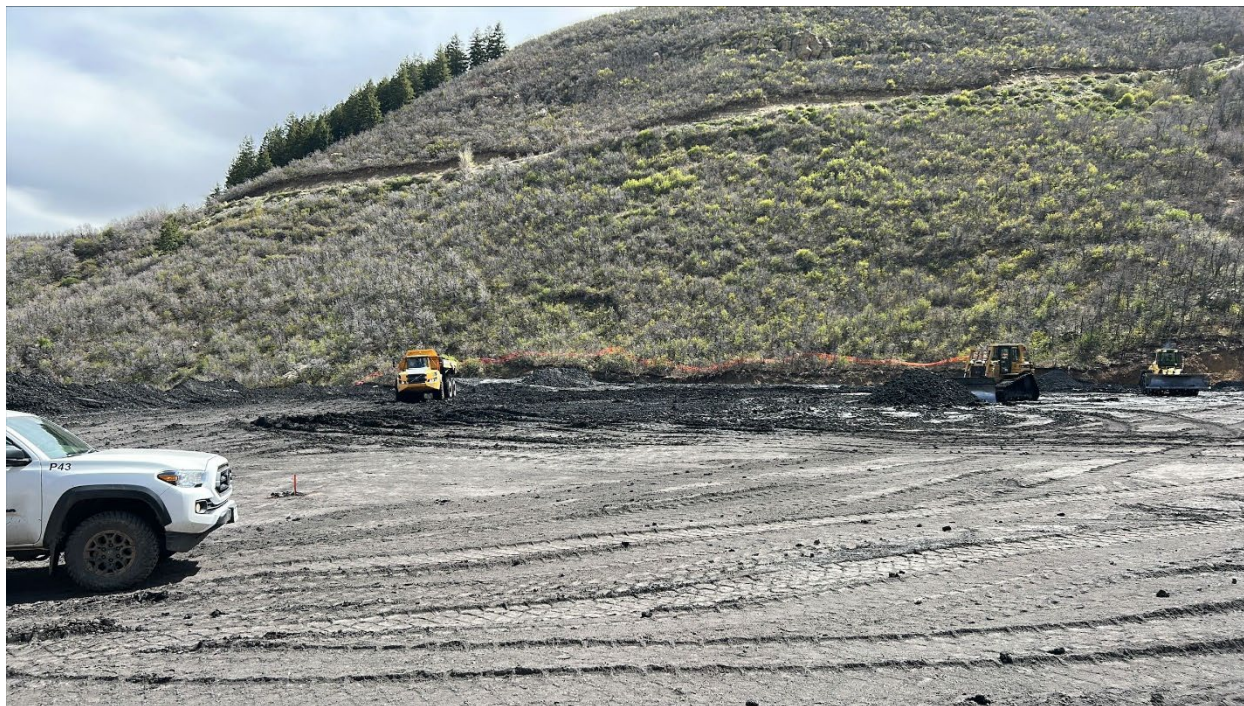
Figure 6: RPEE, showing preliminary compaction with haul truck
