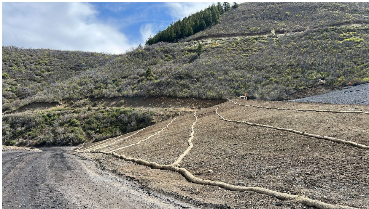
Figure 8: RPEE outslope, showing straw wattles
