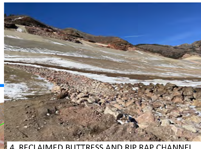
4. RECLAIMED BUTTRESS AND RIP RAP CHANNEL.
