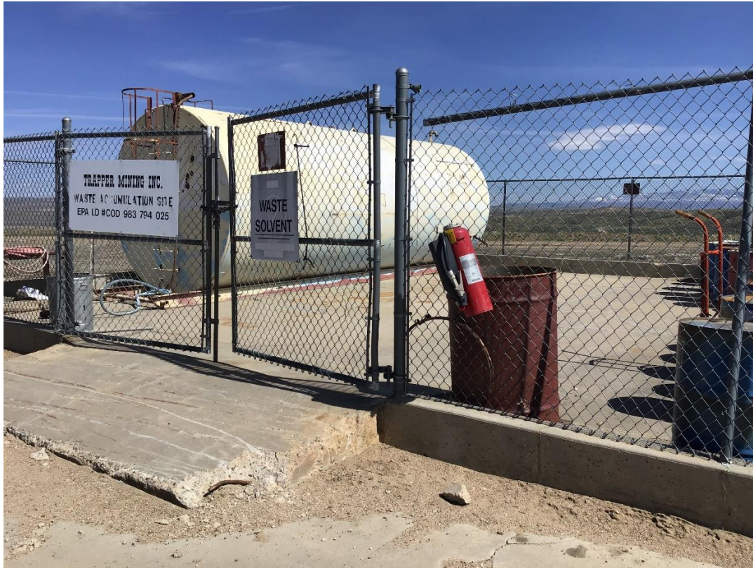
Photo 3: Waste solvent accumulation site, secured with adequate containment.
