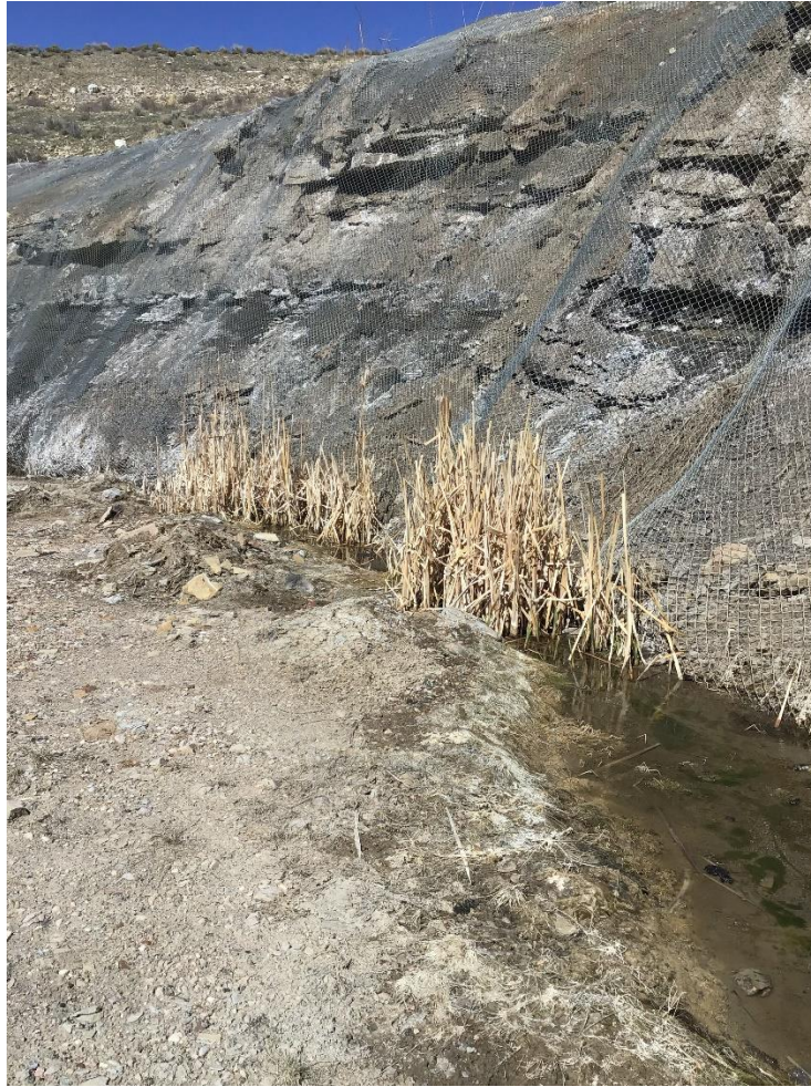
Photo 4: Spoil Spring drainage ditch, flow impeded by cattails.
