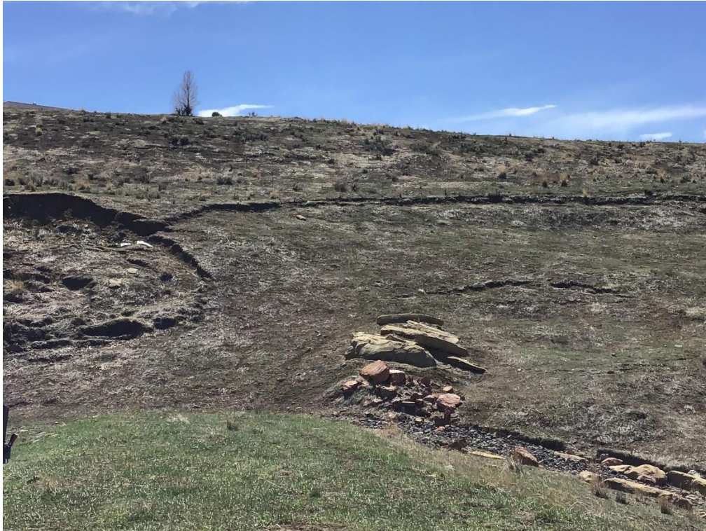
Photo 1: Old Pond 6 slump with crack going across the slope.
