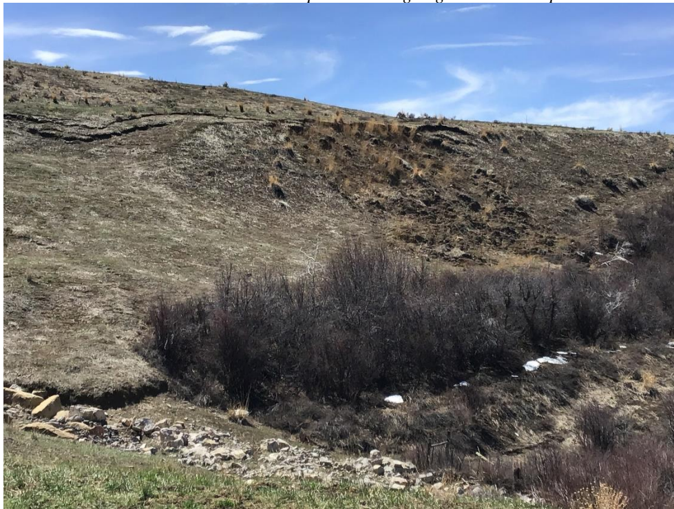
Photo 2: Pond 6 slump of 2023 at the right in the photo and slope fissures.
