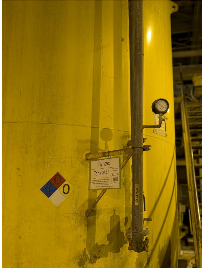
Photo 8: Mill EPF 2.6 - 33,000 gallon Syntex Storage
