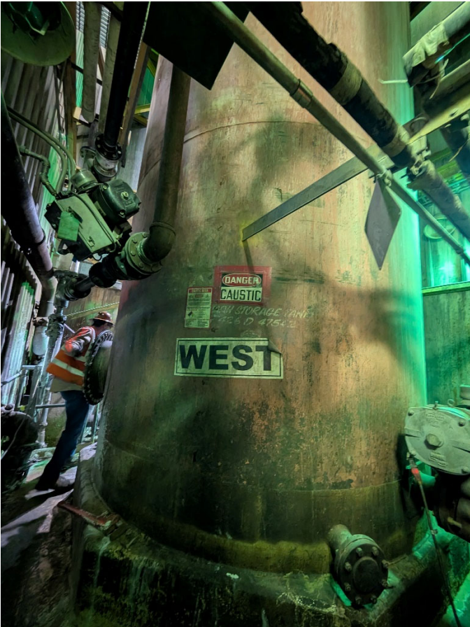
Photo 1: Mill EPF 2.1 - Sodium Hydroxide Storage West Tank in building adjacent to the north side of the Mill.
