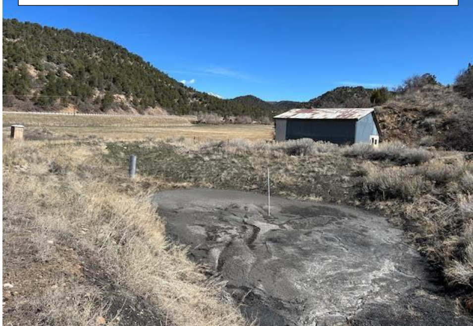
Photo 10: The east sediment pond at King I.
