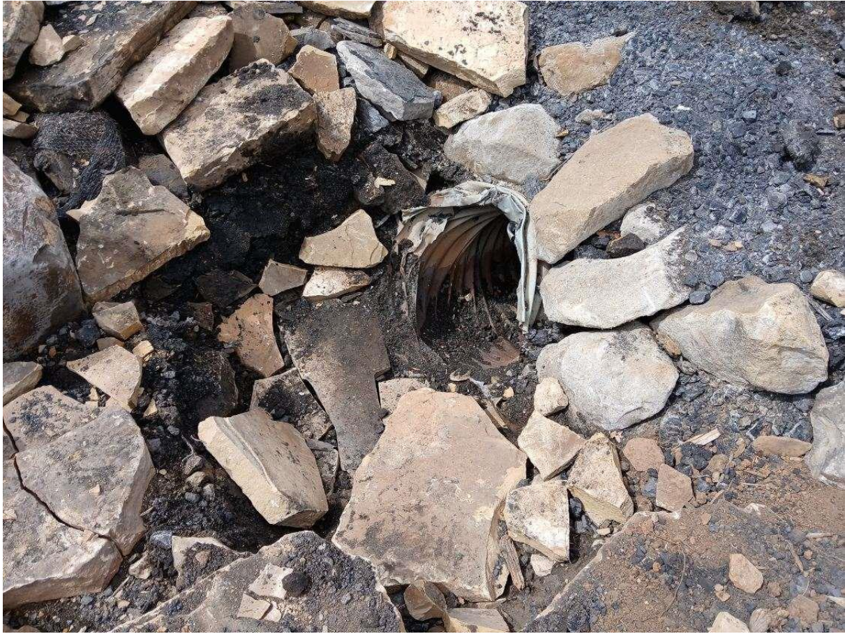
Picture 2: King I Culvert Inlet Cleaned
