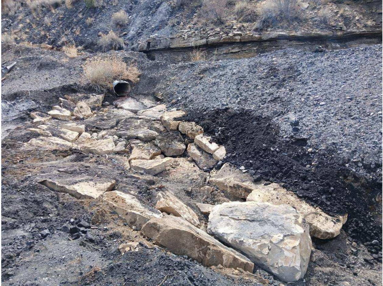
Picture 1: King I Outlet Culvert Cleaned
