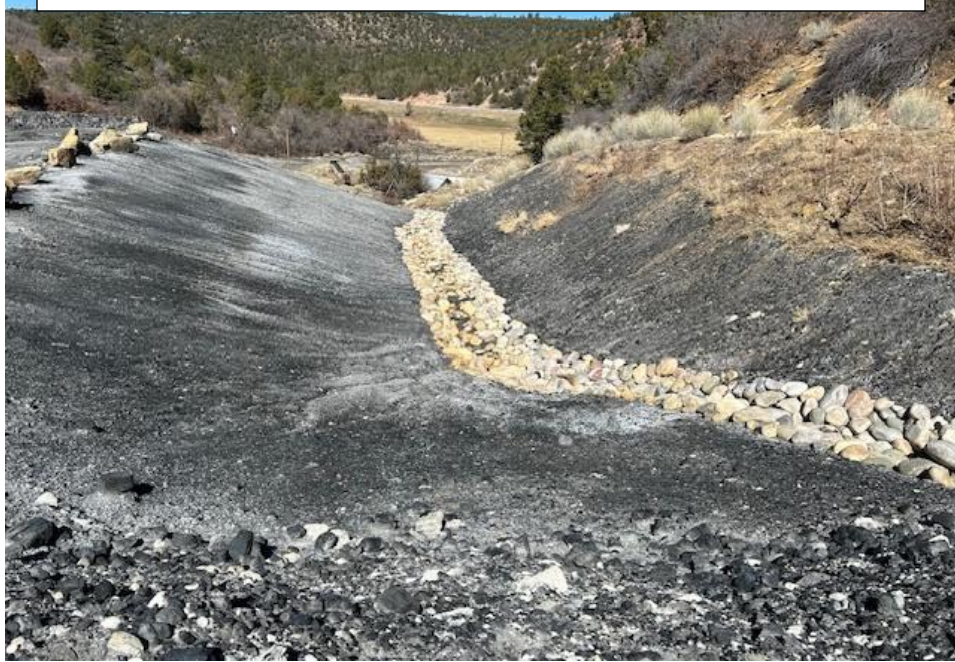
Photo 9: The armored portion of Reach 13.
