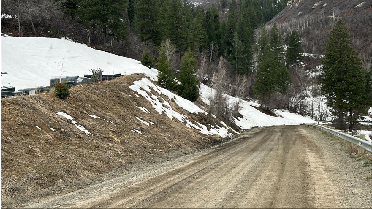
Figure 17: Small slump on edge of Material Storage Area
