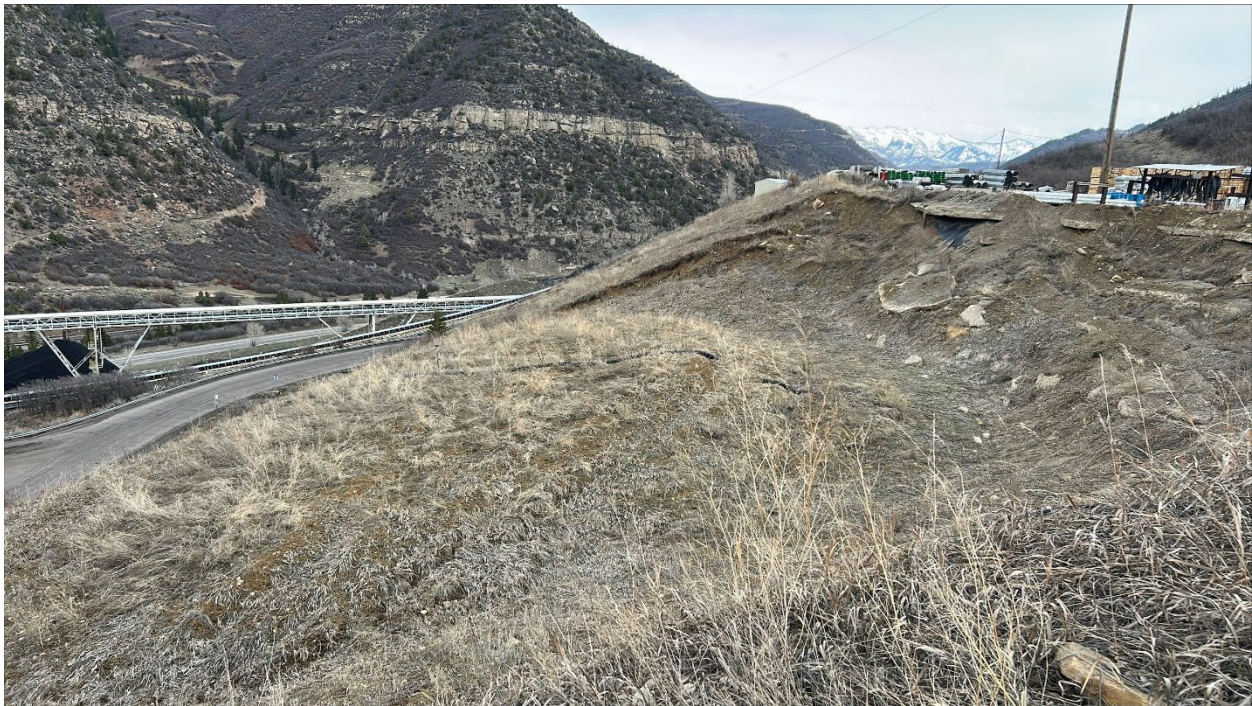
Figure 20: Slump on Material Storage Bench
