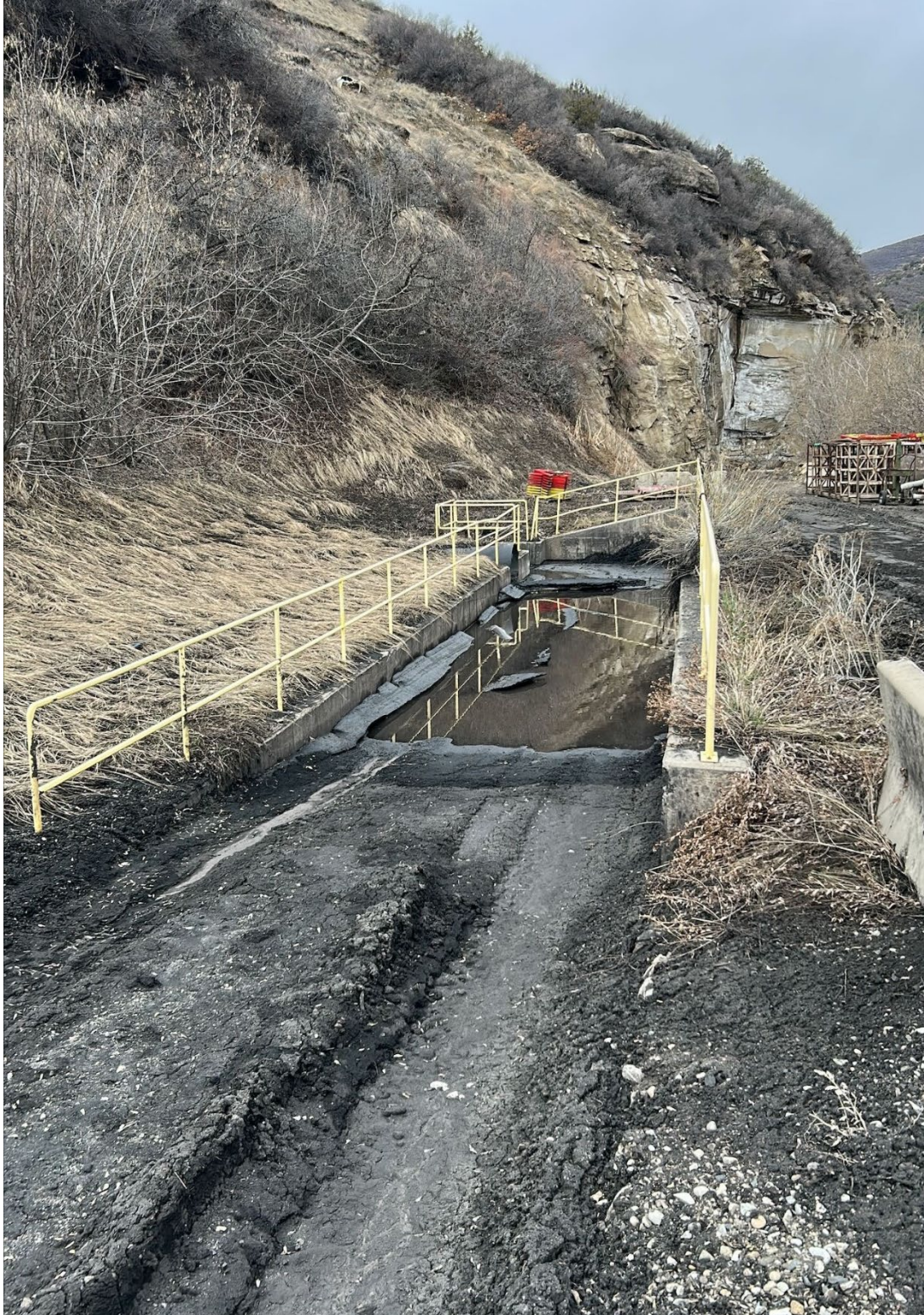
Figure 14: Sediment trap at inlet to C5E-1
