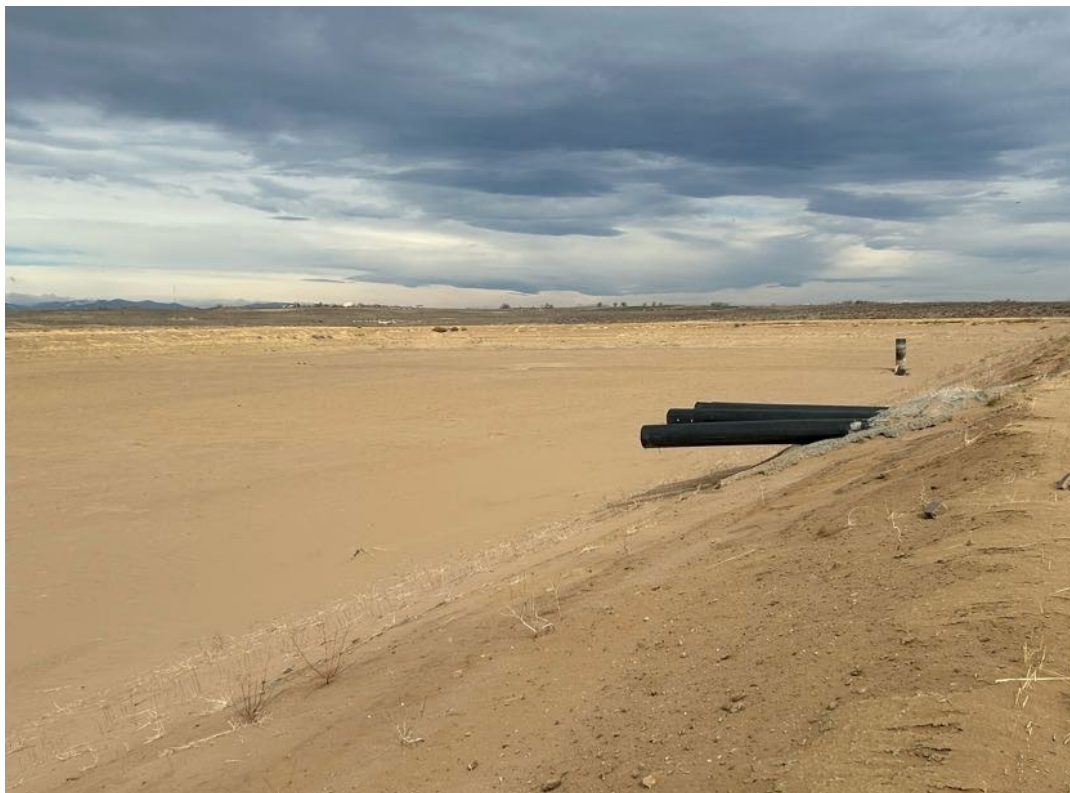
Photo 15: Overflow spillway pipes connecting North Settling Pond 4 and Milton Reservoir, facing north.
