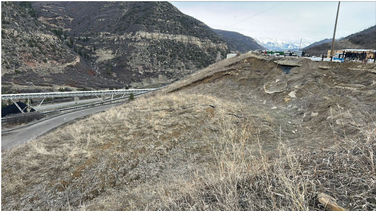
Figure 20: Slump on Material Storage Bench
