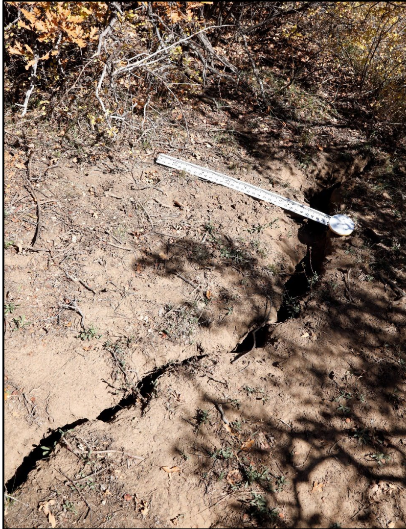
Figure 2: The largest of the cracks observed at Location 2 in fall 2022, south of the across road on Traverse C-C'.
