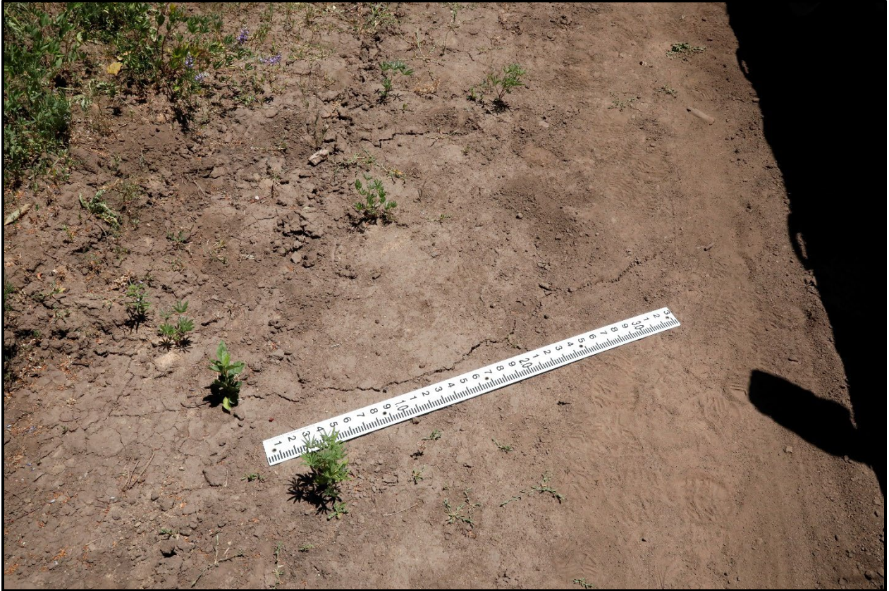
Figure 7: Example of an observed crack along the north side of E-seam Longwall Panel SS3 during spring 2023 site visit
