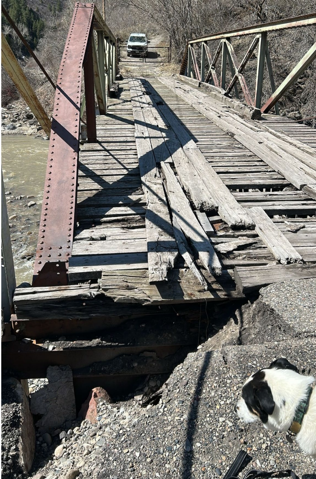
Figure 8: Erosion at edge of bridge, and damaged timber
