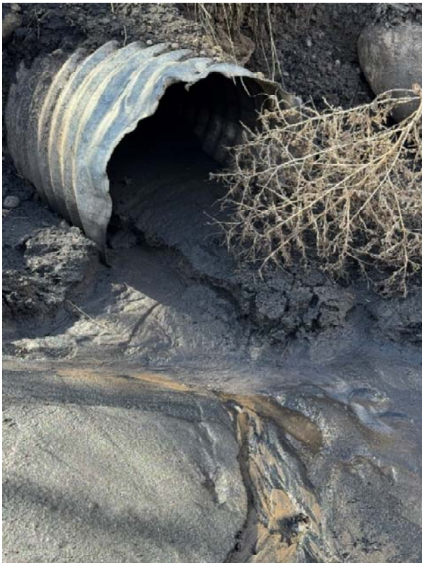
Pic. 6 – Sediment accumulation at the culvert outlet that drains the detention pond (behind scale house).
