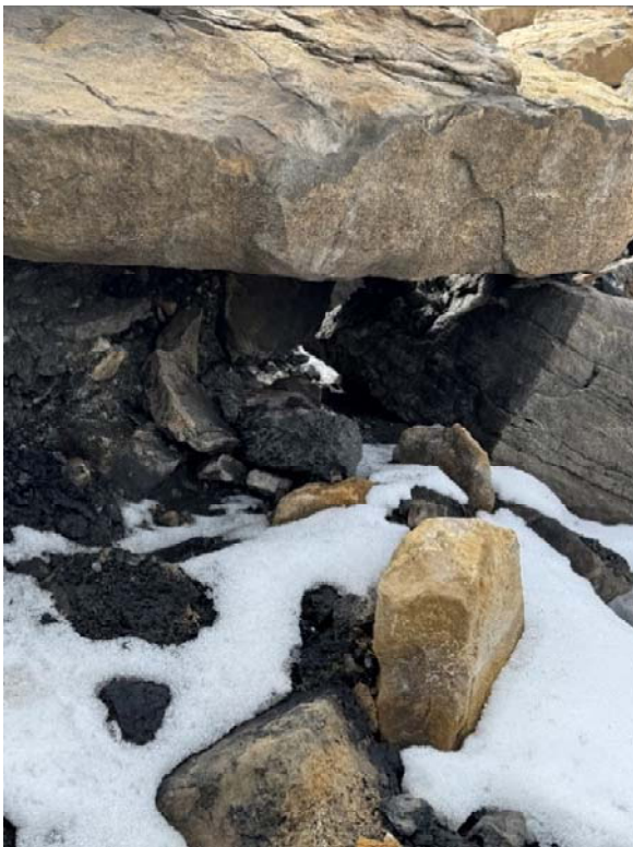
Pic. 2 – Reach 9 (at stilling basin) with voids forming between rock riprap.
