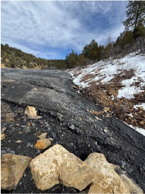
Pic. 5 – Runoff from upper waste pile into Reach 10 showing some erosion and beginning of undercutting at rock armor.
