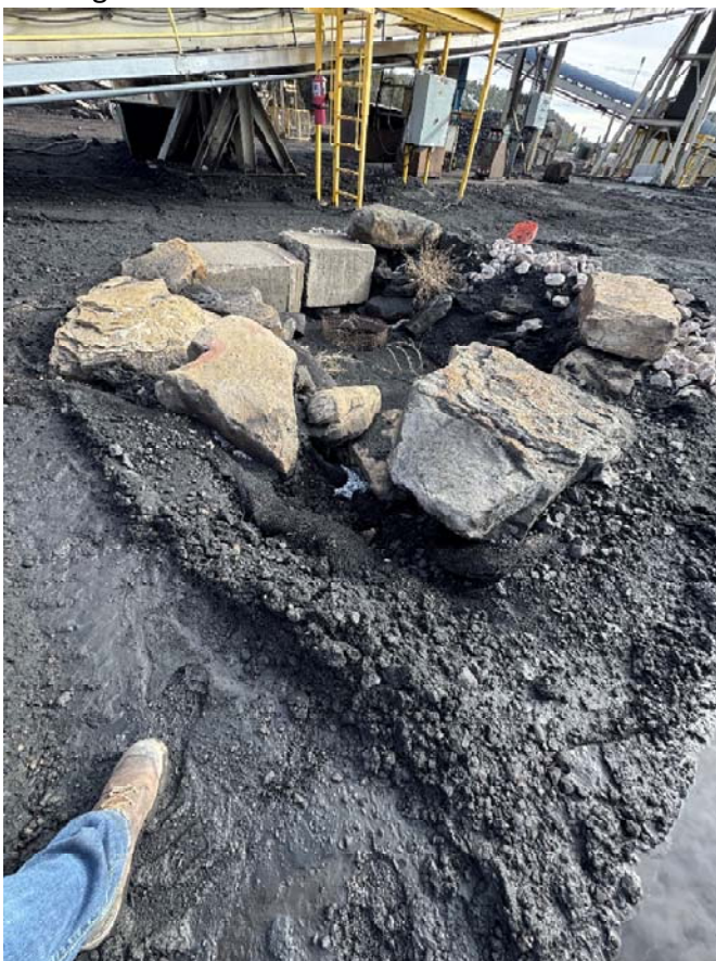
Pic. 4 – Some erosional cutting to drain near conveyor belt.
