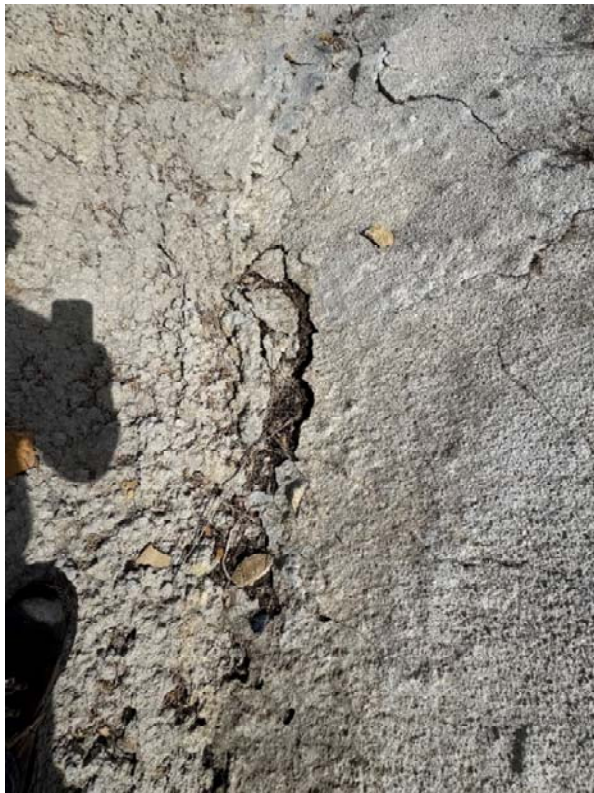
Pic. 7 – Cracking and exposed subsurface in upper armored section of Reach 1.
