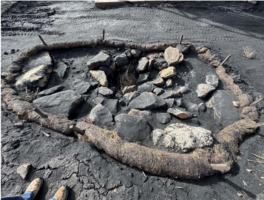
Pic. 5 – Straw wattles and rock armor near the vibratory processing area.
