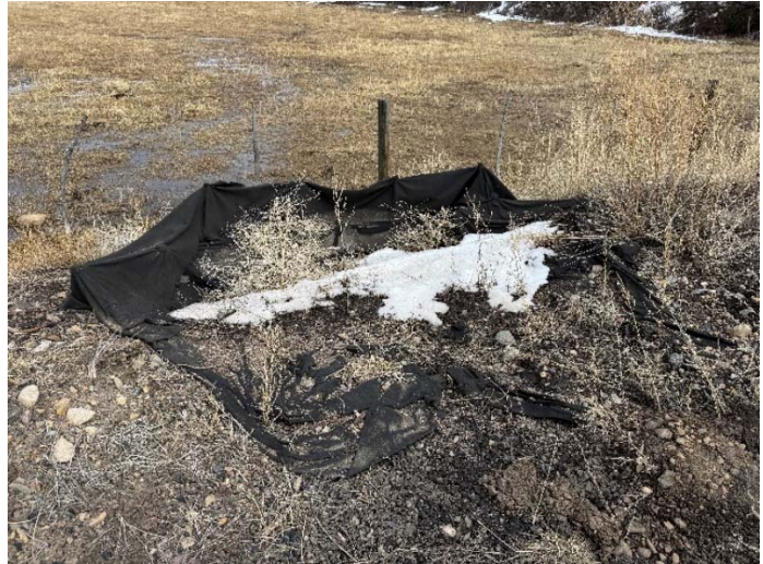
Pic. 1a and 1b – Sedimentation traps in need of dredging and anchoring.
