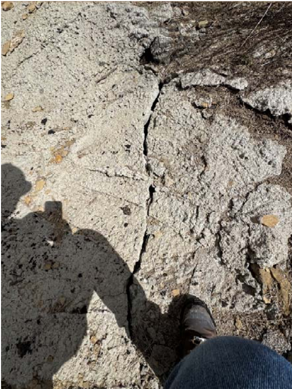
Pic. 6a and 6b – Cracks within lower armored section of Reach 1.
