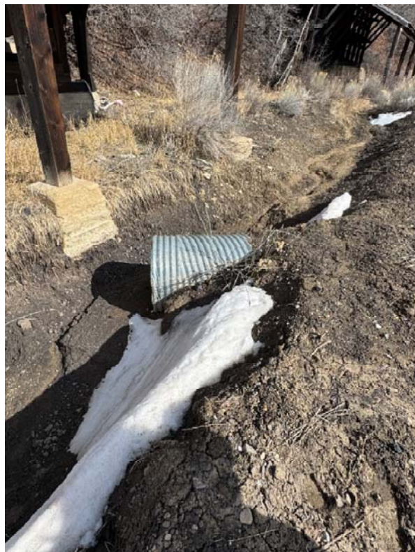
Pic. 8 – Some sediment accumulation at culvert outlet near bottom of Reach 5.
