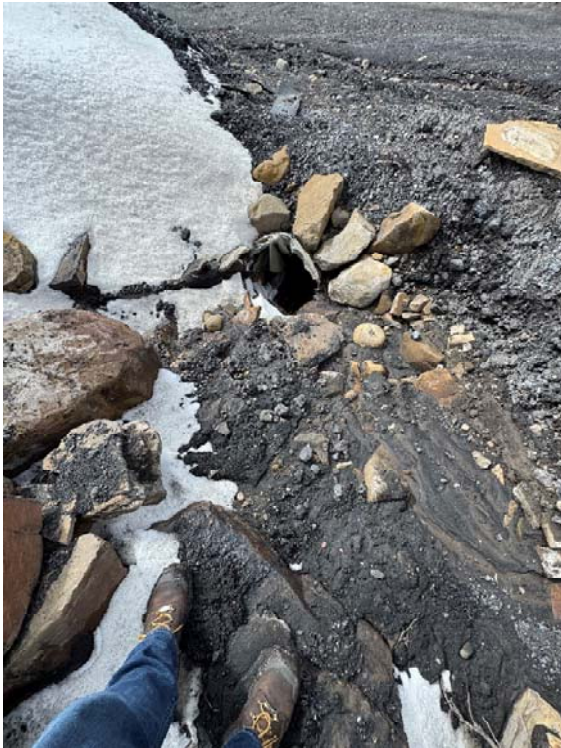
Pic. 3 – Damaged culvert that drains lower Reach 10 under the haul road and into the lower waste pile channel section. Flow does not appear to be impeded.
