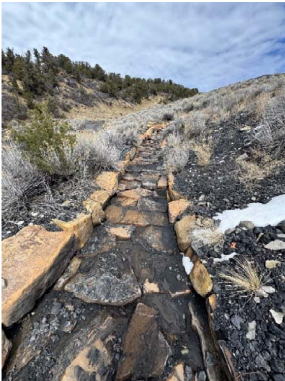
Pic. 4a and 4b – Reach 10, armored sections between upper and lower waste piles.
