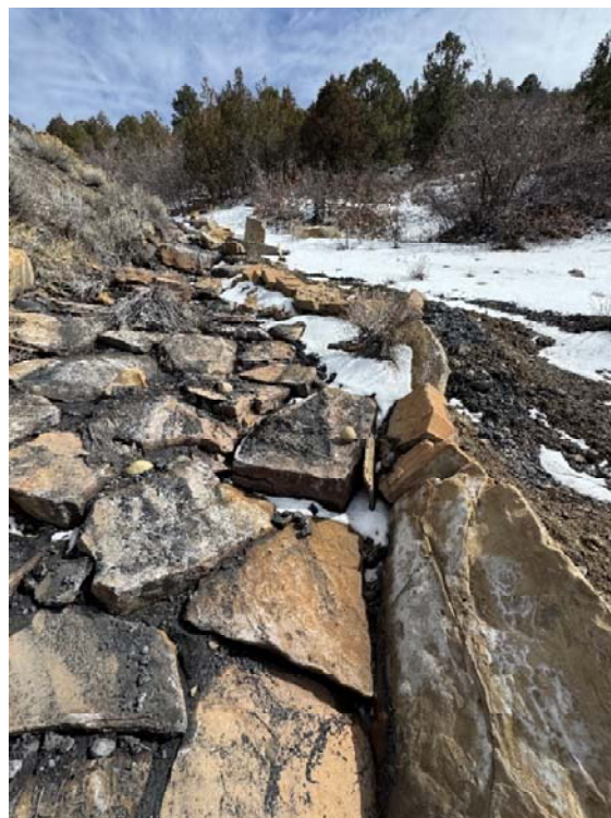
Pic. 4a and 4b – Reach 10, armored sections between upper and lower waste piles.
