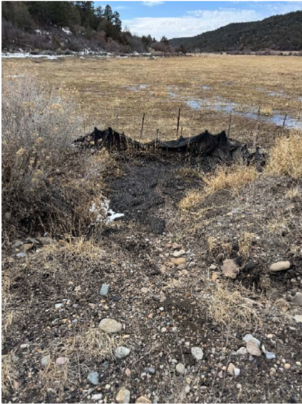
Pic. 1a and 1b – Sedimentation traps in need of dredging and anchoring.
