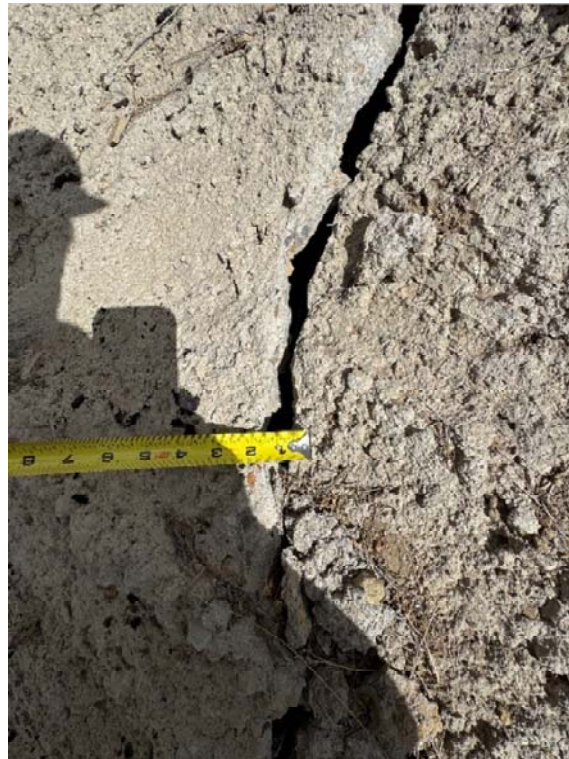
Pic. 6a and 6b – Cracks within lower armored section of Reach 1.
