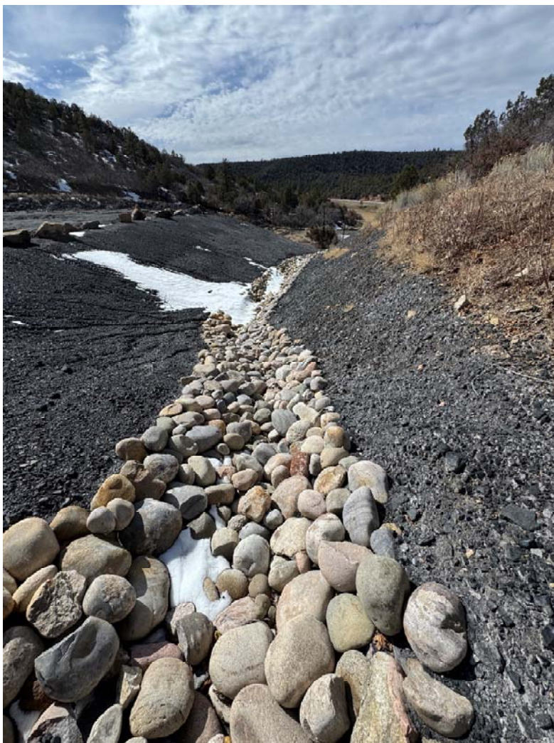
Pic. 4 – Drainage off the lower waste pile into rock riprap is generally good condition.
