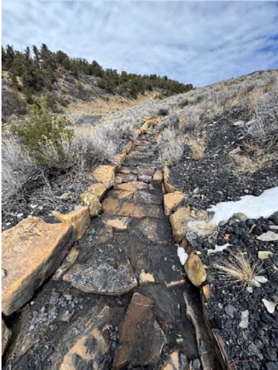
Pic. 1a and 1b – Reach 10, riprap between upper and lower waste piles, preventing escape of runoff.
