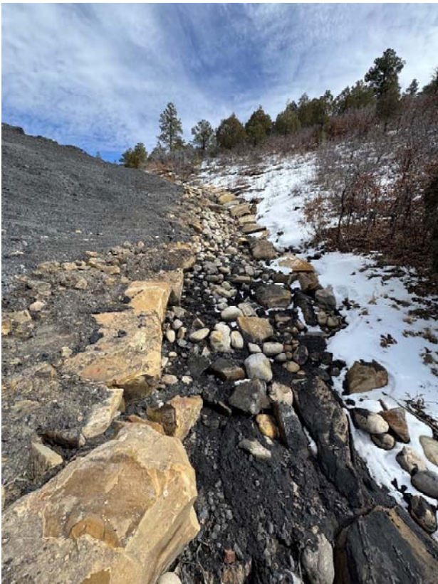
Pic. 2 – Reach 10, upper section channel riprap functioning as intended.
