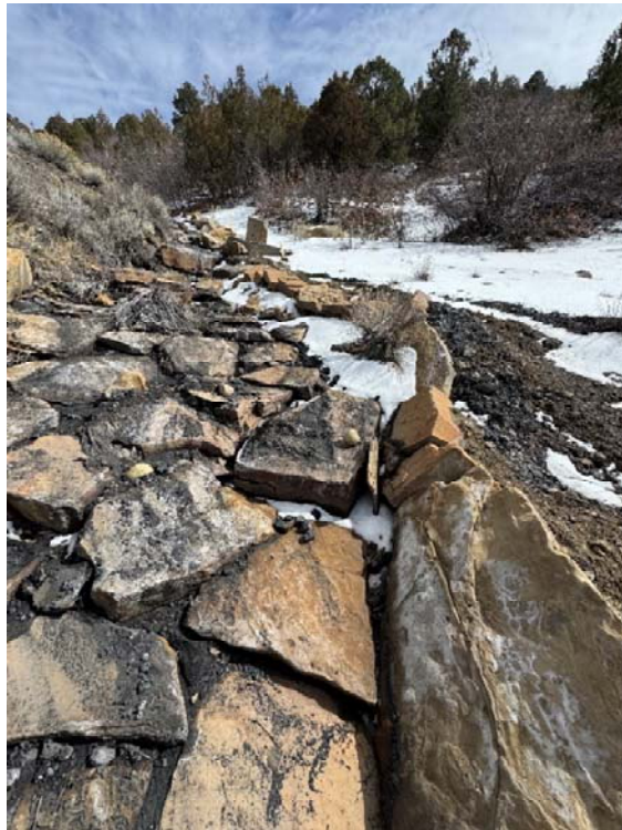
Pic. 1a and 1b – Reach 10, riprap between upper and lower waste piles, preventing escape of runoff.
