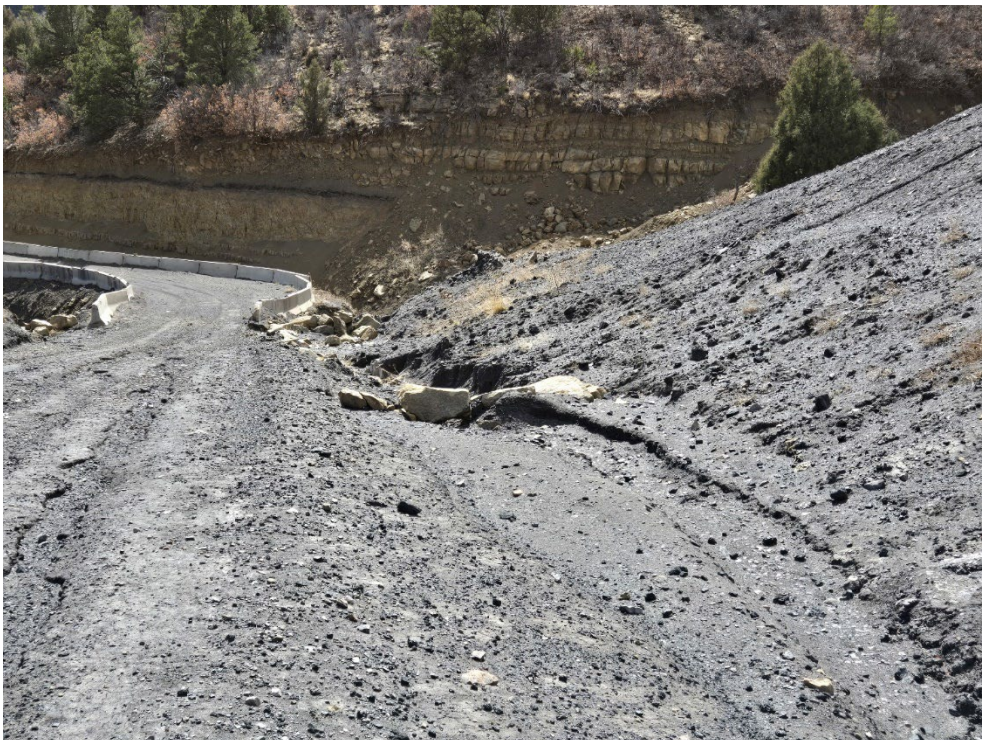
Photo 16: Looking along the ditch on the north side of the RDA road, at the toe of the most recently placed slope where check dams have been undercut.
