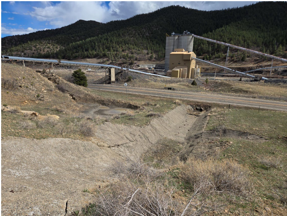
Photo 2: Containment Area no. 5 and the emergency spillway for Pond 08.
