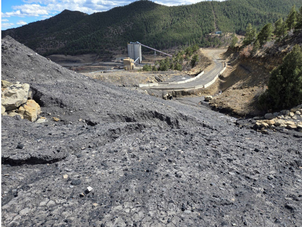
Photo 11: Looking at where the top of the RDA is eroding into the unnamed ditch east of ditch D55 leads to C81.
