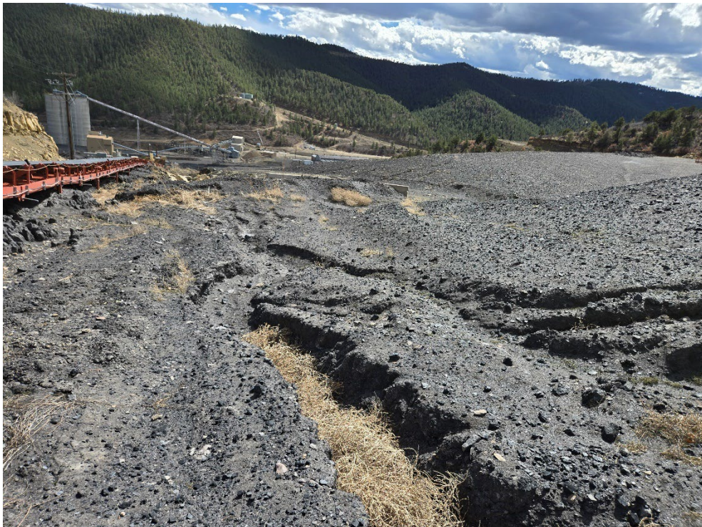
Photo 18: Looking at the erosion running along the west side of the conveyor belt.
