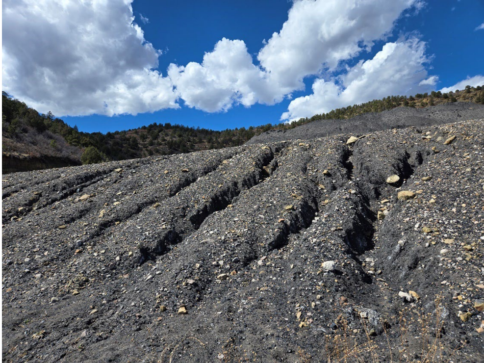
Photo 19: Erosion rills on the south-facing side of the first unreclaimed slope.
