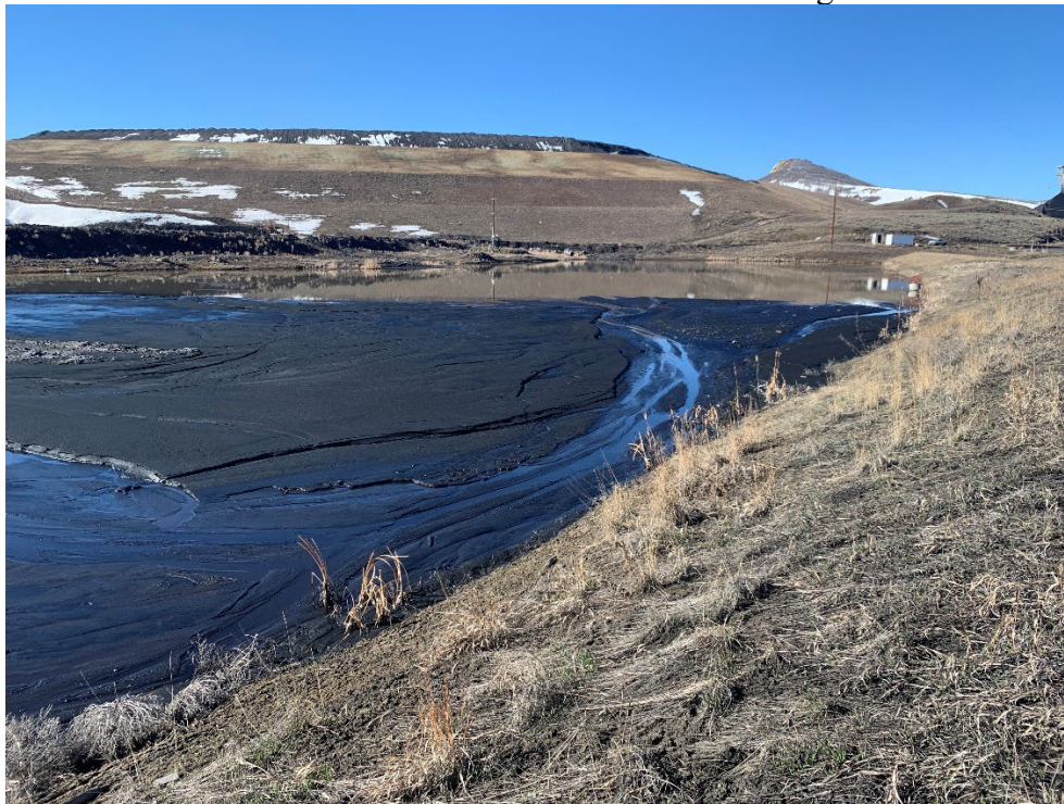
Photo-3 Sediment build up in D-pond
