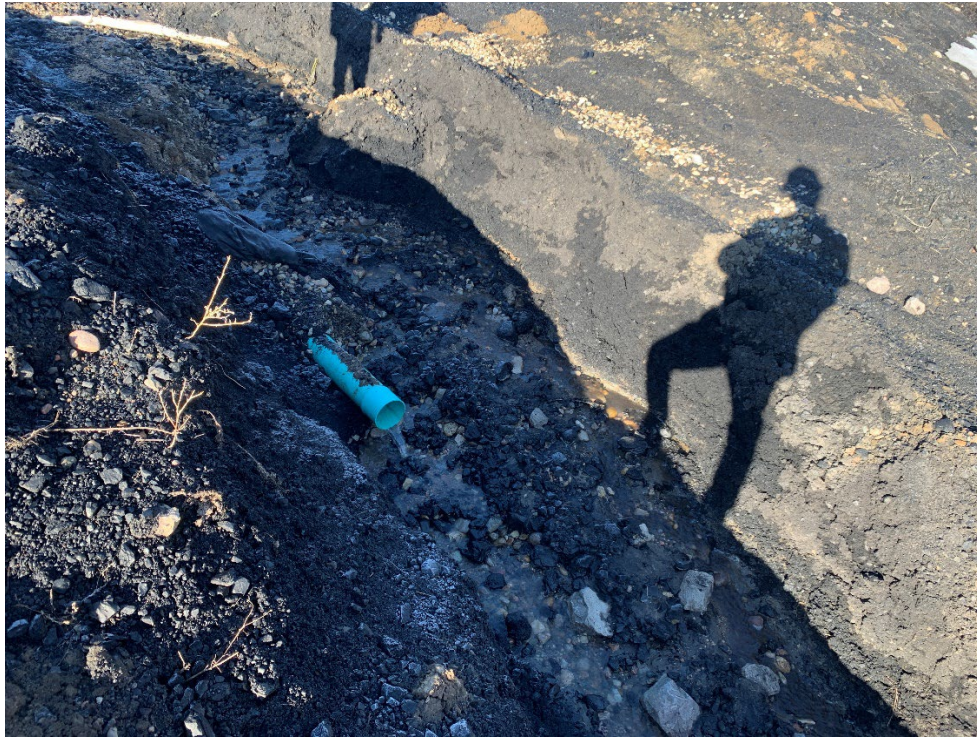
Photo 2- Belt-out-back underdrain discharge
