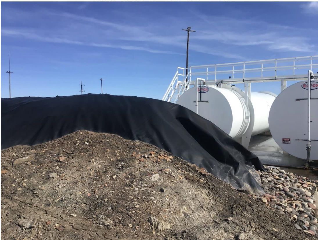
Photo 7: Three 50,000 gallon diesel fuel tanks showing lined containment berm.
