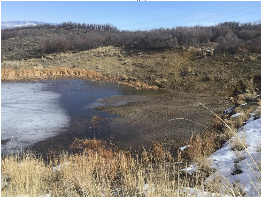
Photo 5: Inlet sediment fan in East Middle Flume #1 Pond.
