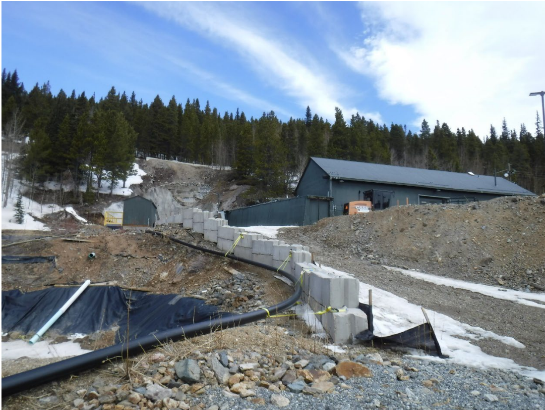
Photo 5: Pipeline conveying effluent water to Pond 1. Heat tape in the pipeline prevent freezing.
