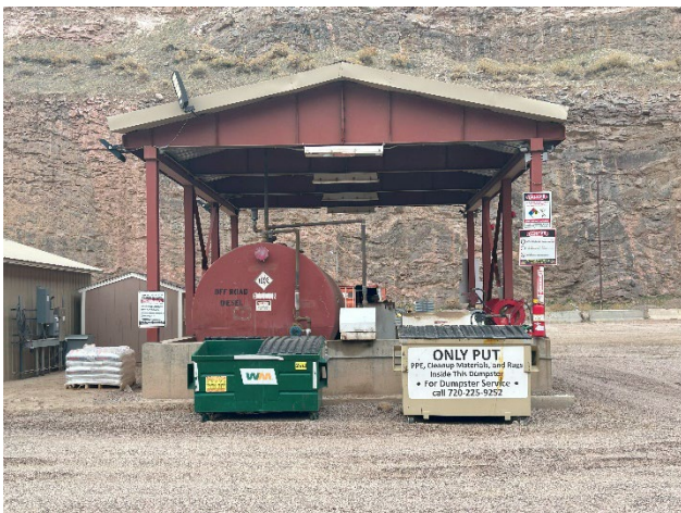
Photo 5: Fuel storage area. Note the double lined containment area.
