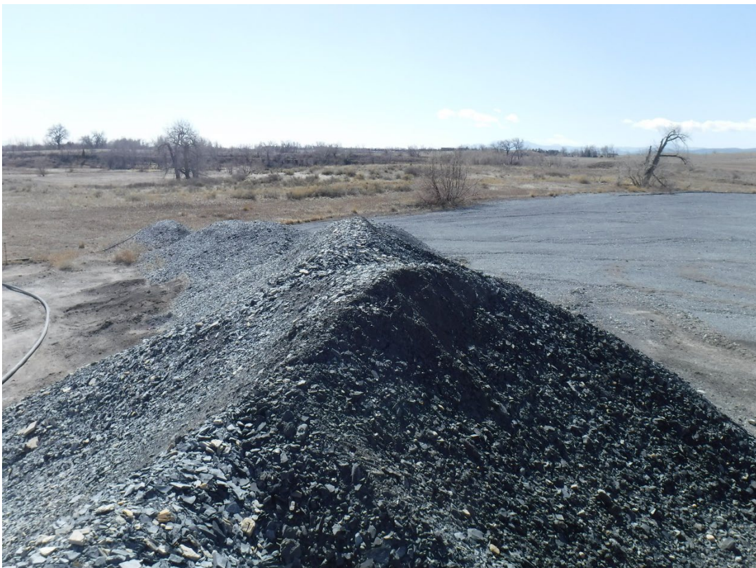
Photo 10: Shale cover material along edge of exposed CKD
