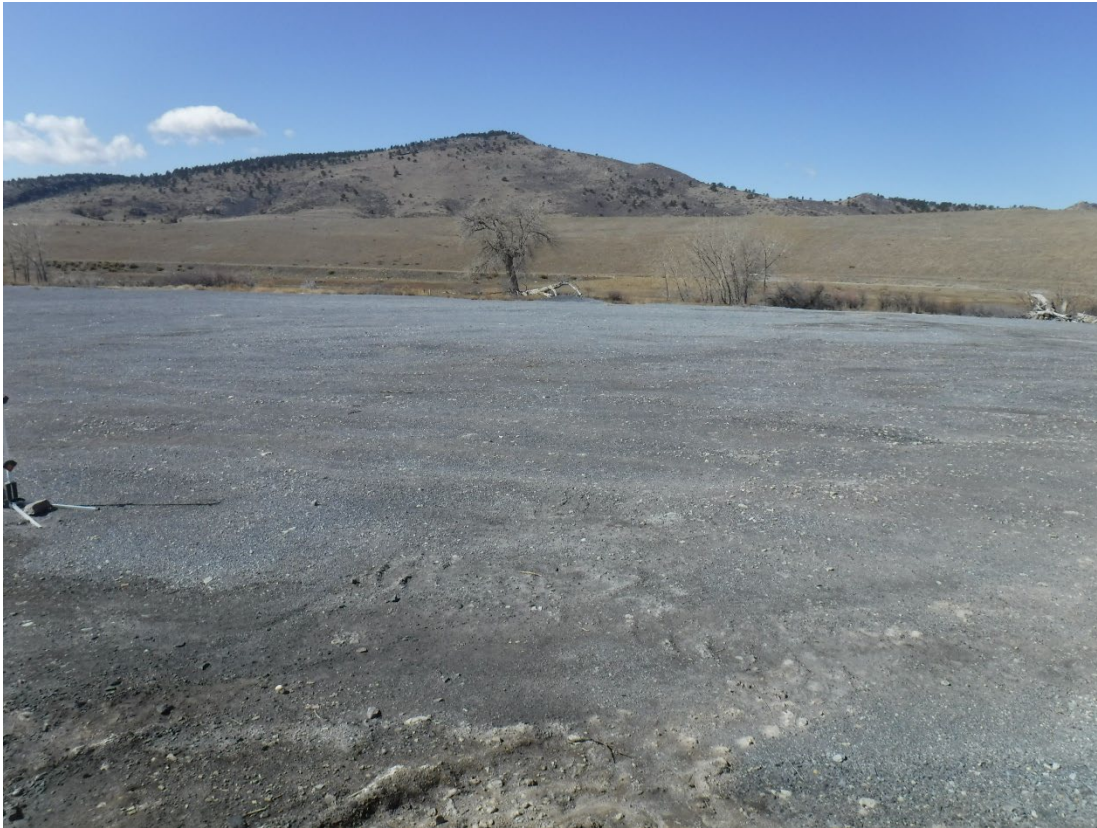
Photo 11: Shale cover material spread over CKD material, looking west
