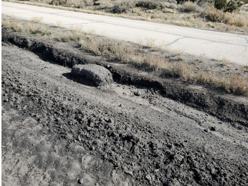
Photo 15 – View to the north of haul road drainage ditch with hay bale.
