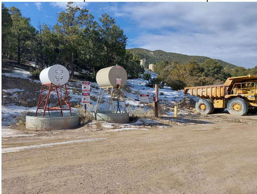
Photo #12: Fuel tanks with secondary storage.
