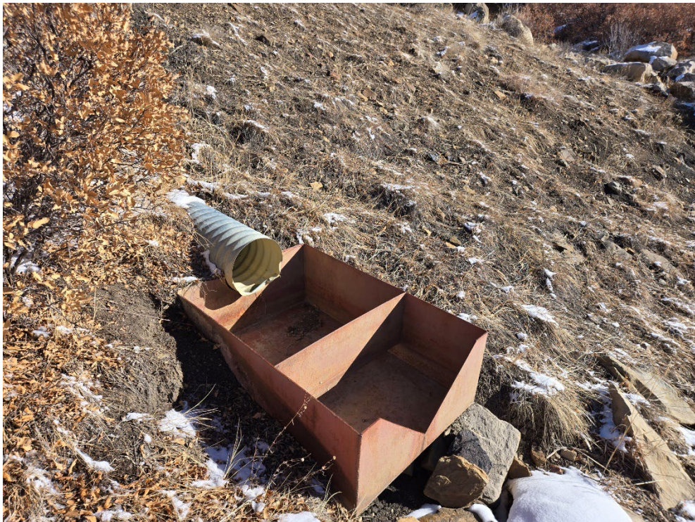
Photo 6: Flume for Pond 007a.
