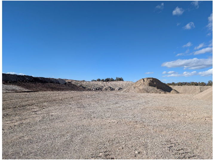
Mined areas graded to 2H:1V
