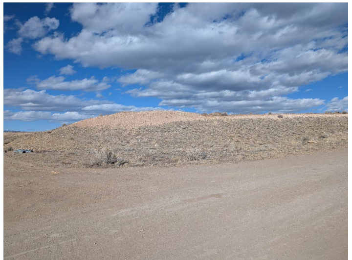
Mined areas graded to 2H:1V
