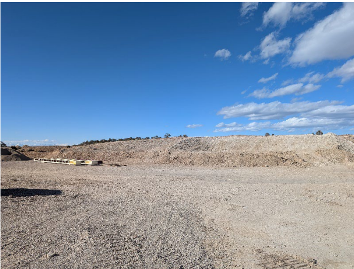
Mined areas graded to 2H:1V
