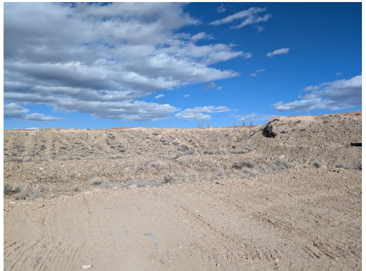
Mined areas graded to 2H:1V
