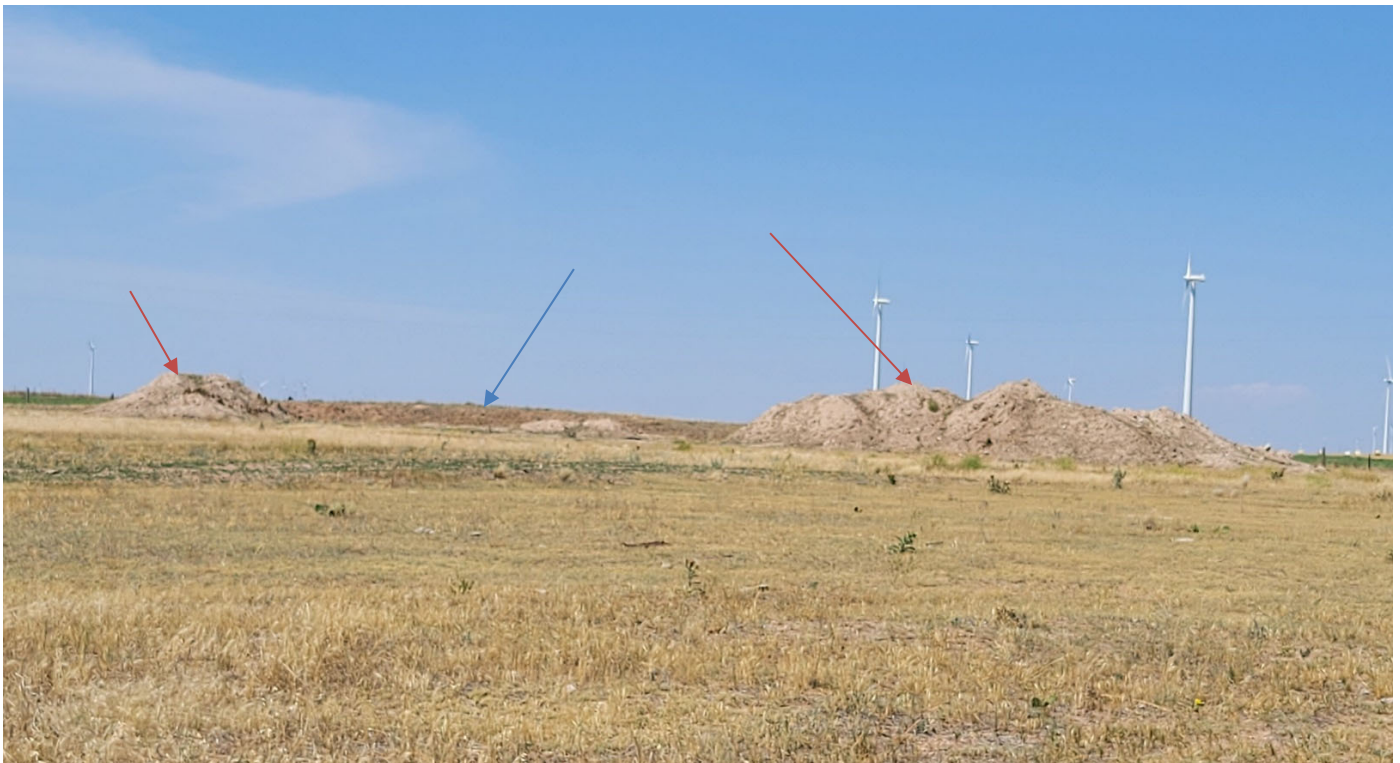
Blue arrow points to topsoil stockpile along western boundary of the permit area. Red arrows point to fill material to be used for future reclamation.
