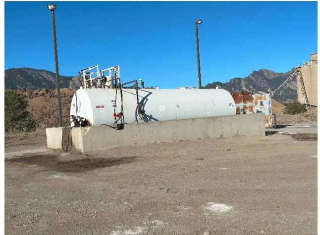
Photo 4: Double-lined fuel storage near processign area.
