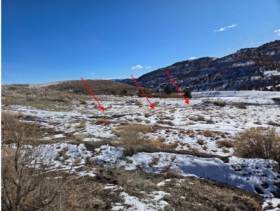
Photo 3: Looking southeast toward Pond 006A from the base of the Reclaimed Area Above Pond 006A. The arrows point to where erosion has cut across the road and entered into the ditch with check dams (see Photo 5).
