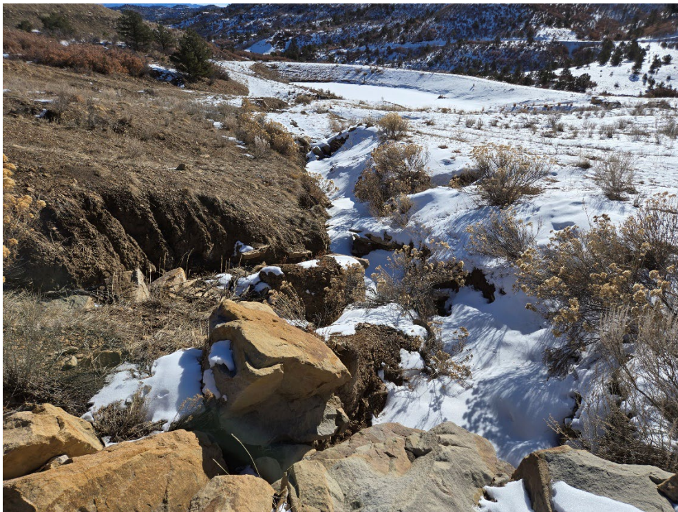
Photo 6: Looking east along where ditches D64, D8, and D7 converge. The check dams in this area need to be repaired and are no longer functioning as designed.
