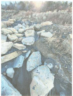
Pic. 4 – Some erosion at stilling basin at base of Reach 10.
