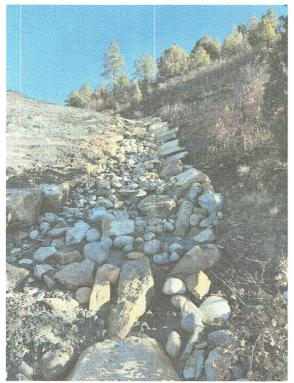
Pic. 1 – Reach 10 upper section channel repair completed.
