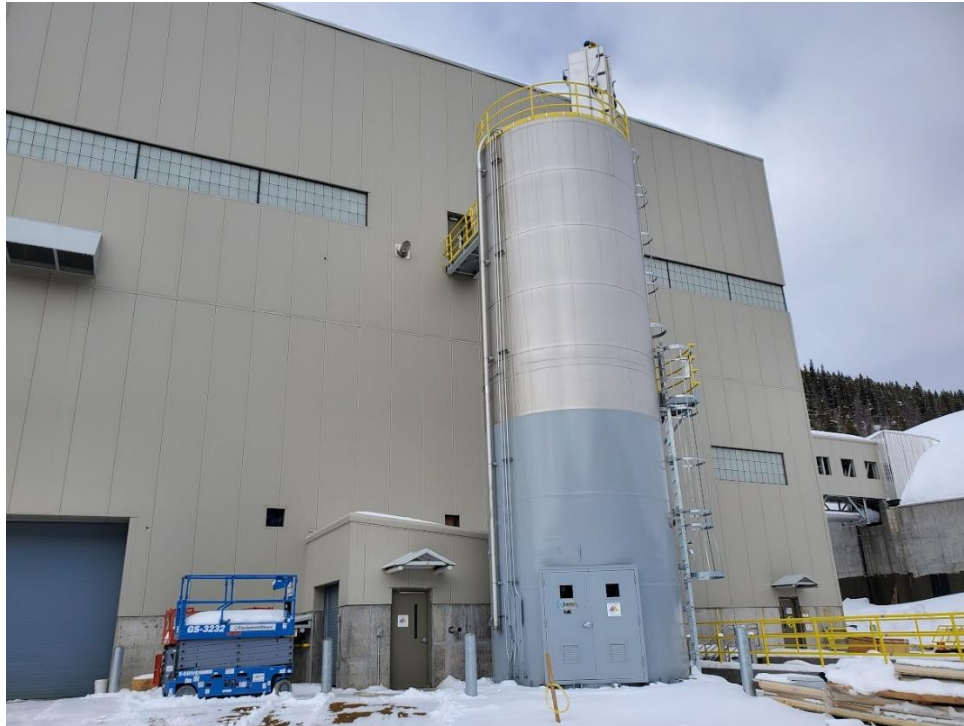
Photo 5 – View to the west of Ferric Sulfide silo outside the MRWTP.
