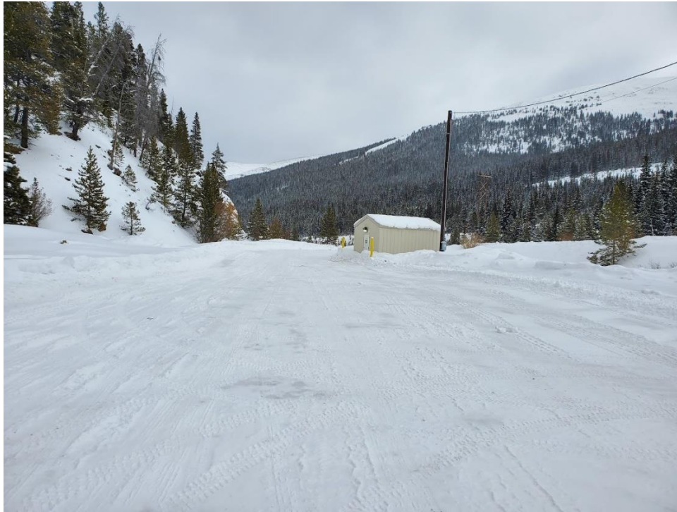
Photo 3 – View to the northeast of area where tailings material was pooled near the access road to the base of 5 Dam.
