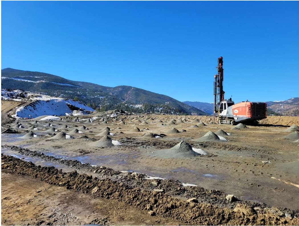
Photo 17: Equipment drilling holes for blasting.
