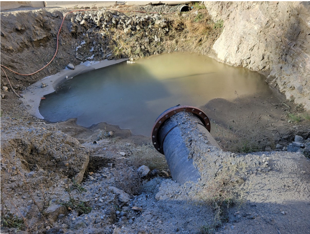
Photo 4: Stormwater retention pond near the entrance to the mine, adjacent to the processing plant.
