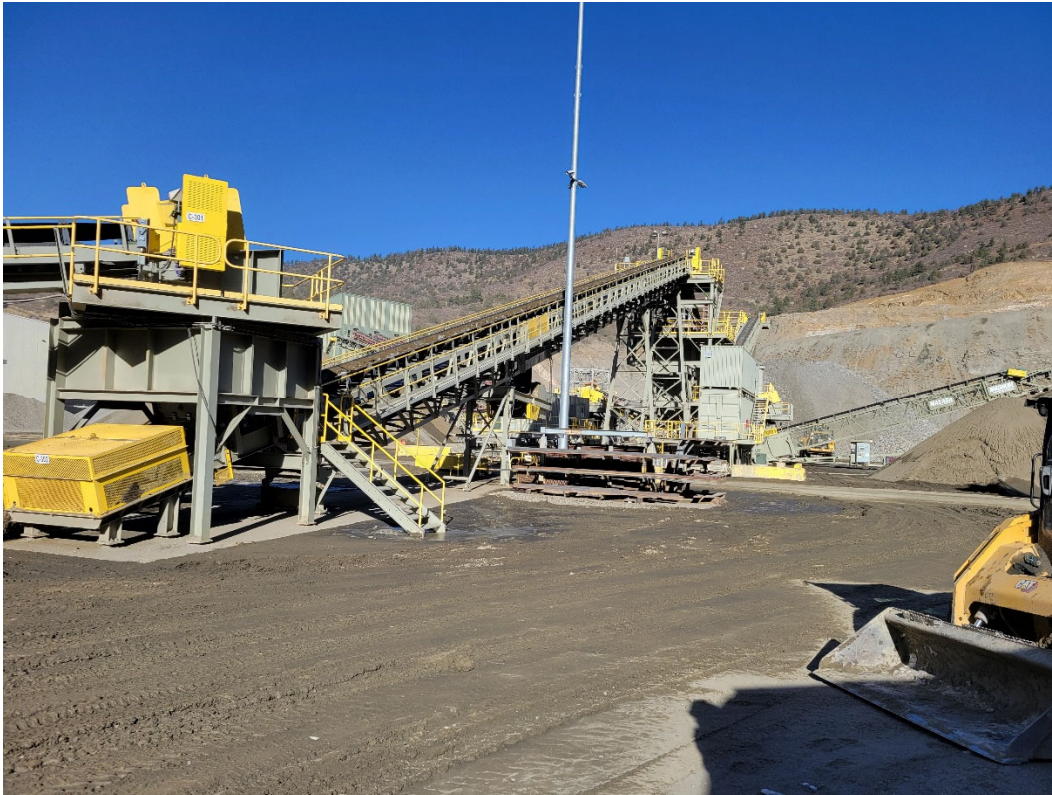
Photo 7: Processing equipment on the floor of the quarry.
