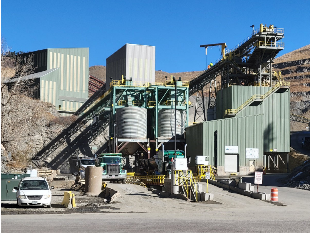
Photo 1: Looking north at the processing facility from the mine office.
