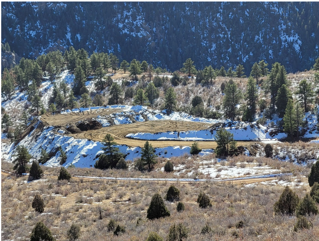
Photo 14: Looking at recently constructed haul road and topsoil storage area in the Spur Amendment Area, on the east side of the permit area.
