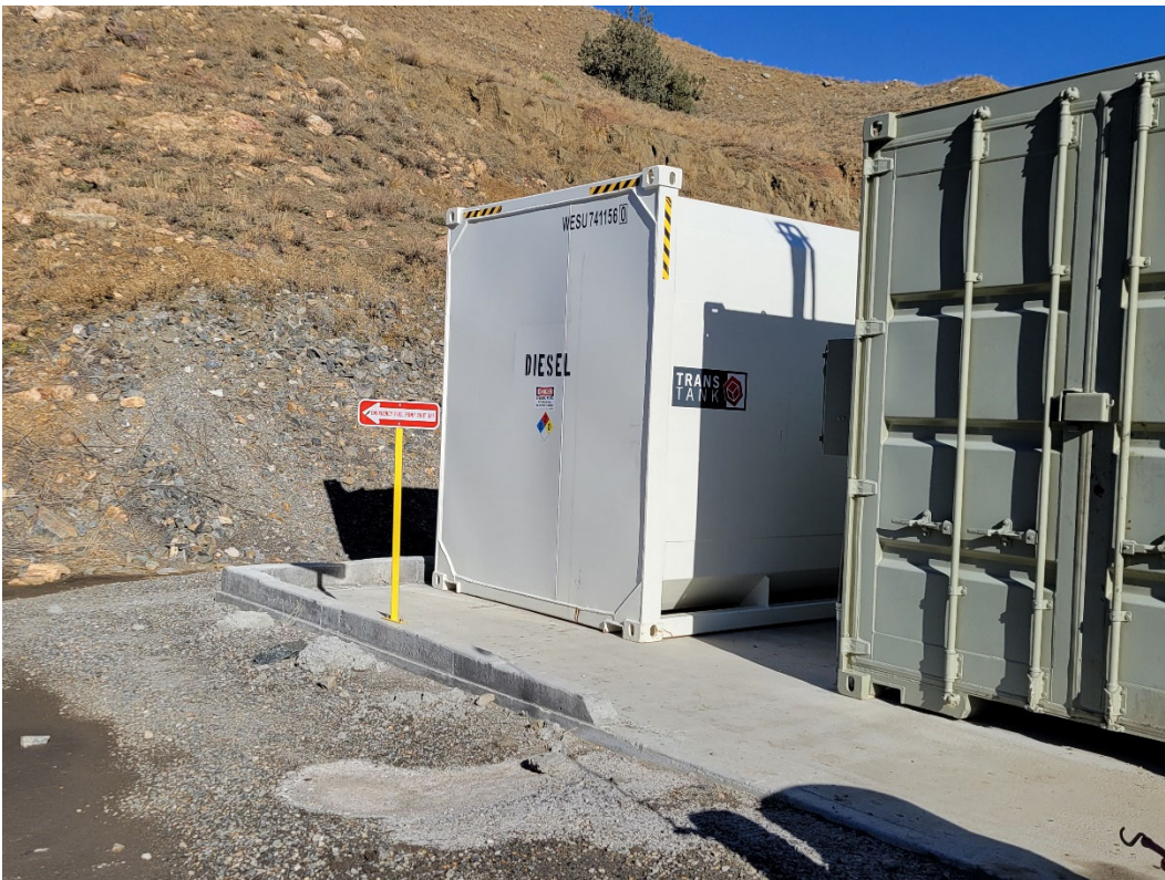
Photo 8: Diesel containment and lubricant storage adjacent to the employee building on level 4 of the quarry.
