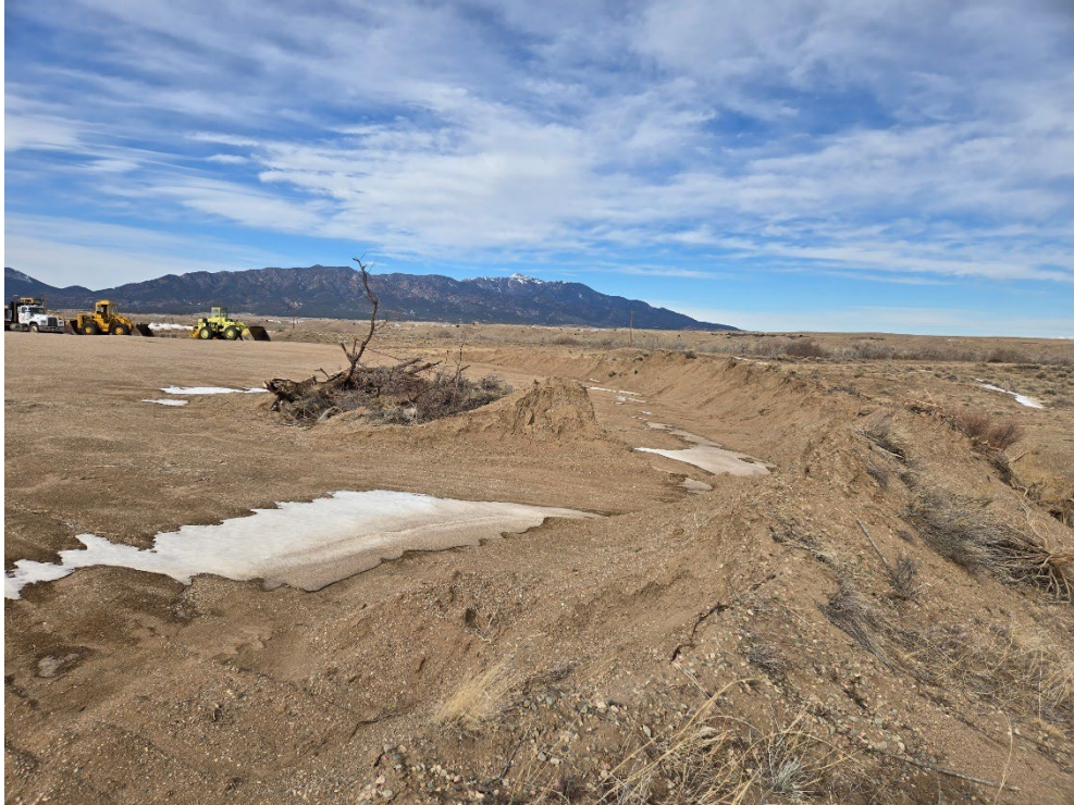
Photo 11: Looking north along the west edge of the remaining Reject Pile. To the west of the remaining pile, there is what appears to be an equipment storage area with the landowner's equipment.
