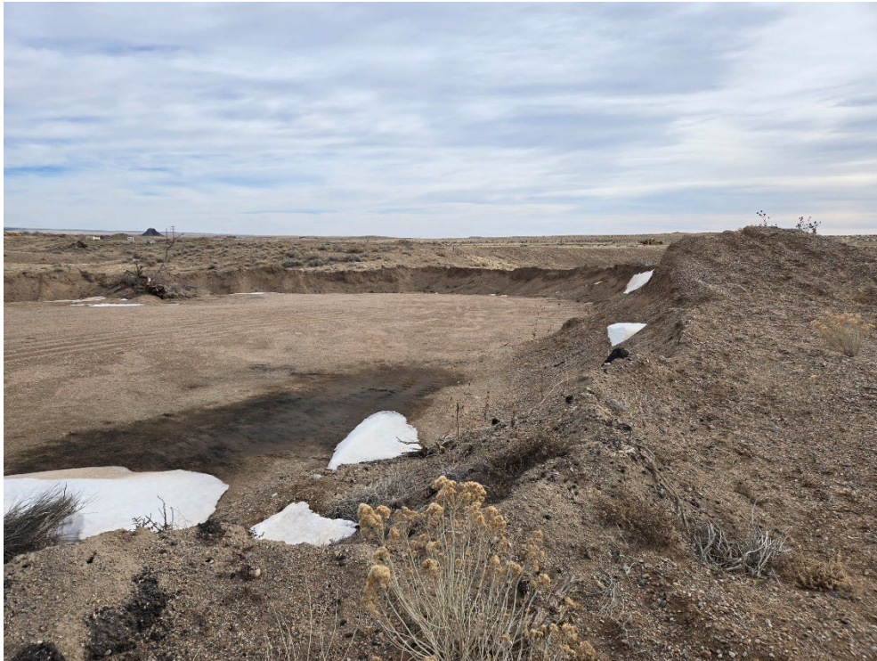
Photo 13: Looking southeast at the spill within the Reject Pile area.
