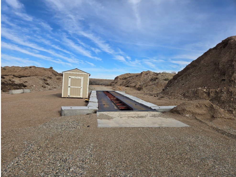
Photo 14: Looking north at the new truck scale and scale house constructed in 2023.
