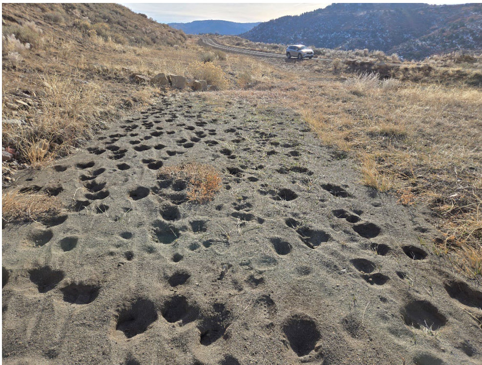
Photo 8: Looking towards the end of D5 (basin area), at the excess amount of sediment deposited within D5.
