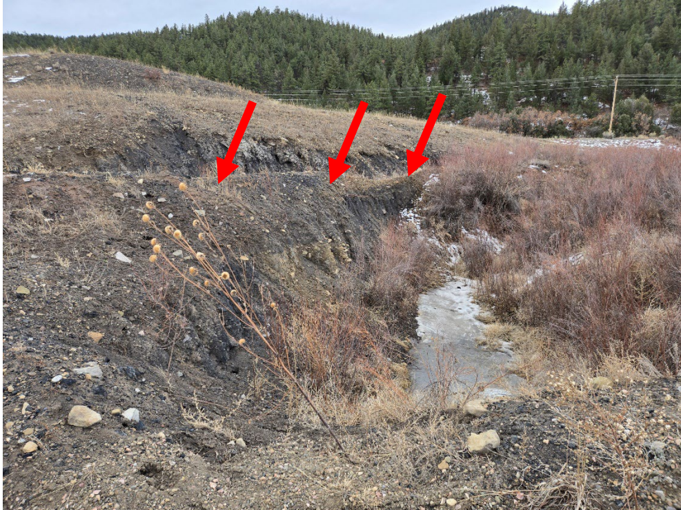
Photo 19: The arrows point to the diversion berm between the clean water and the affected water ditches.
