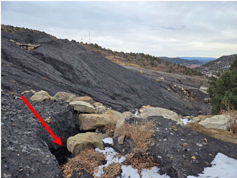
Photo 22: Looking southeast from within the unnamed ditch at the damaged check dam. The arrow points to a hole where water and sediment has run through.
