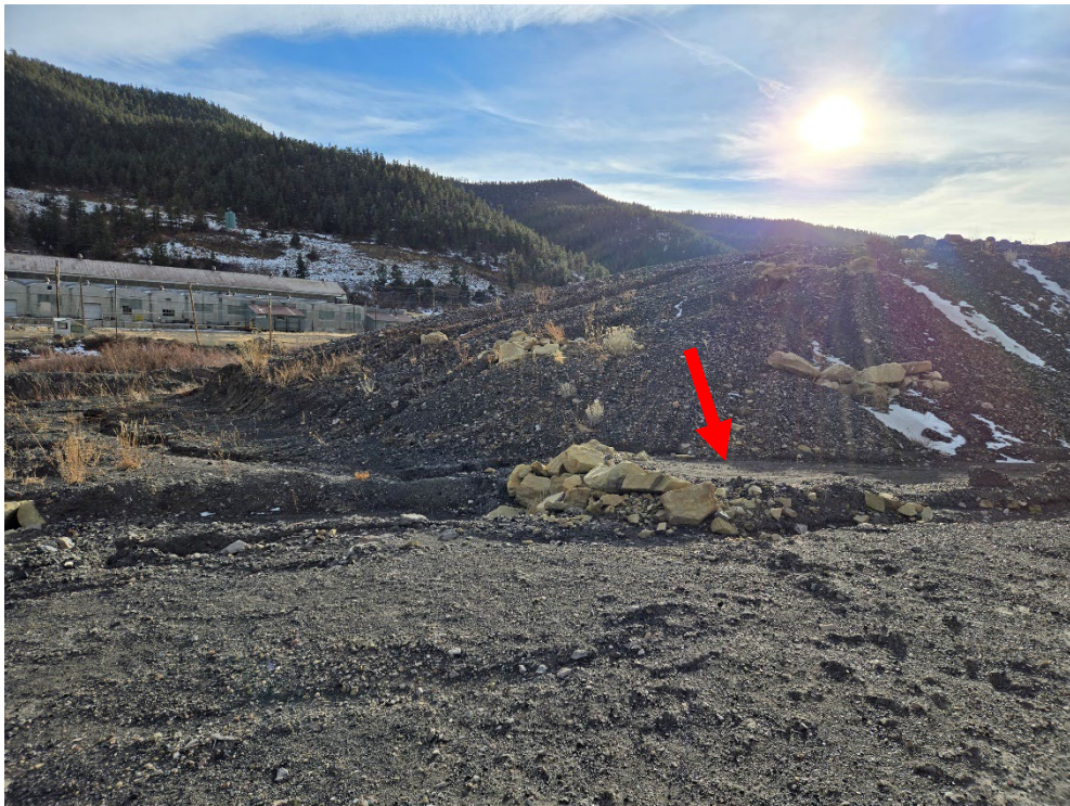
Photo 2: Check dam full of sediment on NE side of DWDA #2 pile.
