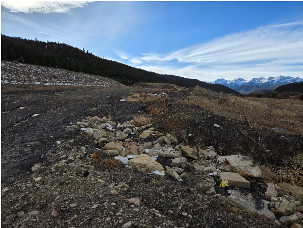
Photo 18: Looking southwest at the check dams along the northside of the subsoil storage area that have begun to fill with sediment.
