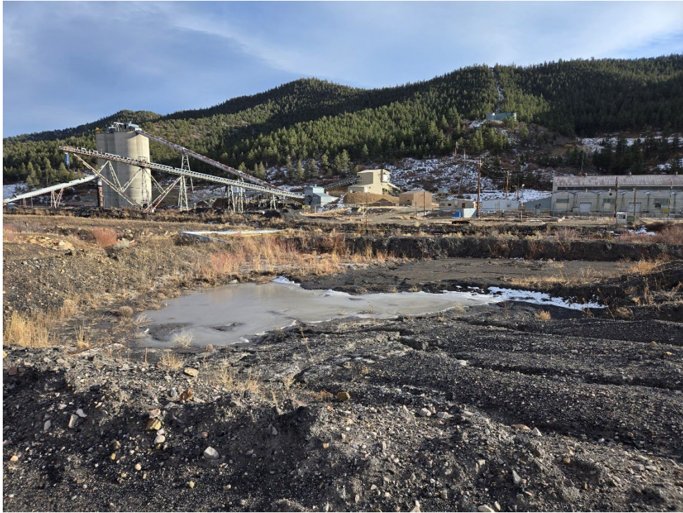
Photo 1: Sediment containment basin, SE corner of DWDA #2.
