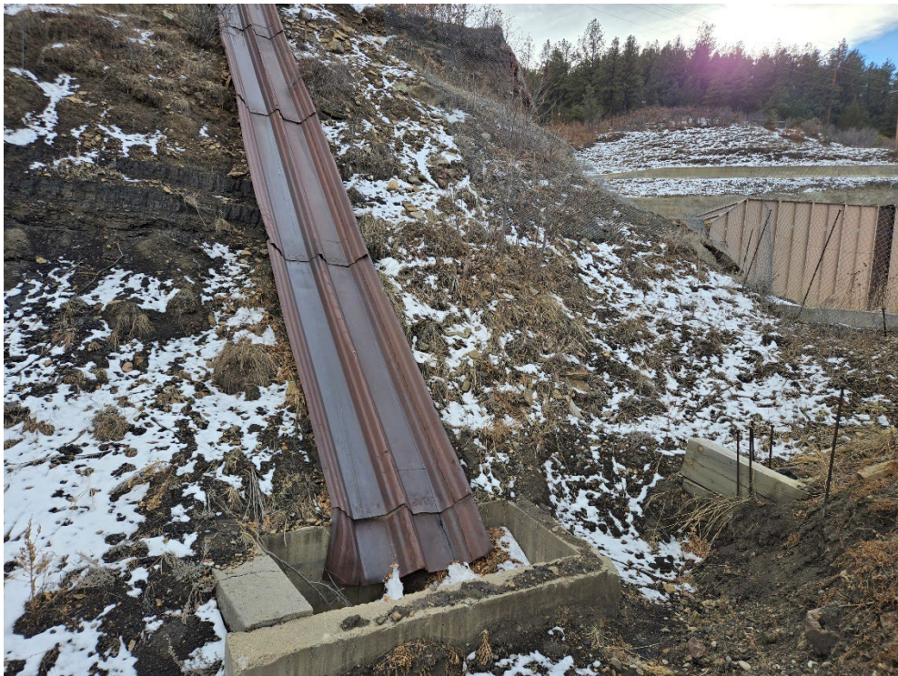
Photo 20: Flume and surrounding concrete and earthen berm structures separating the clean water in D26 from the affected water in D24E.
