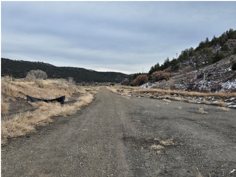
Photo 14: Looking east at the silt fences on the north and south sides of the road leading to Pond 007a, within the S.A.E.
