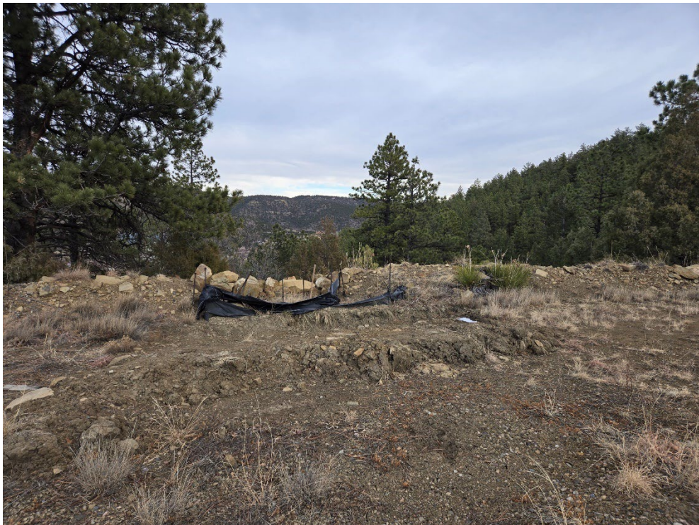
Photo 16: Silt fence along the east side of the S.A.E on the southside of the permit, east of the water tanks.
