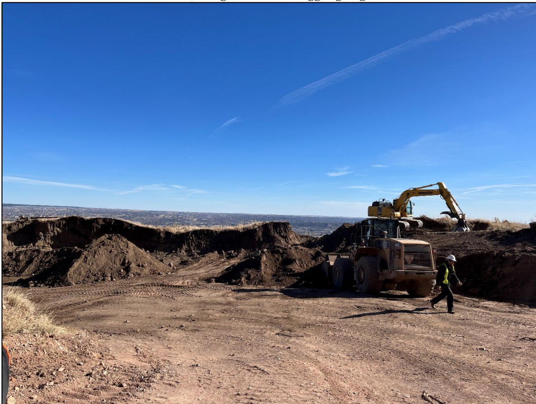
Photo 4: Topsoil stockpiles are being excavated and utilized for road obliteration on USFS land.
