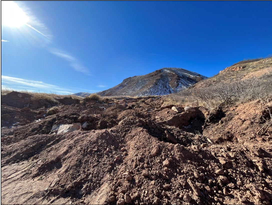
Photo 5: The USFS has approved the rough, pocketed 'design' of the road for the purposes of obliteration.
