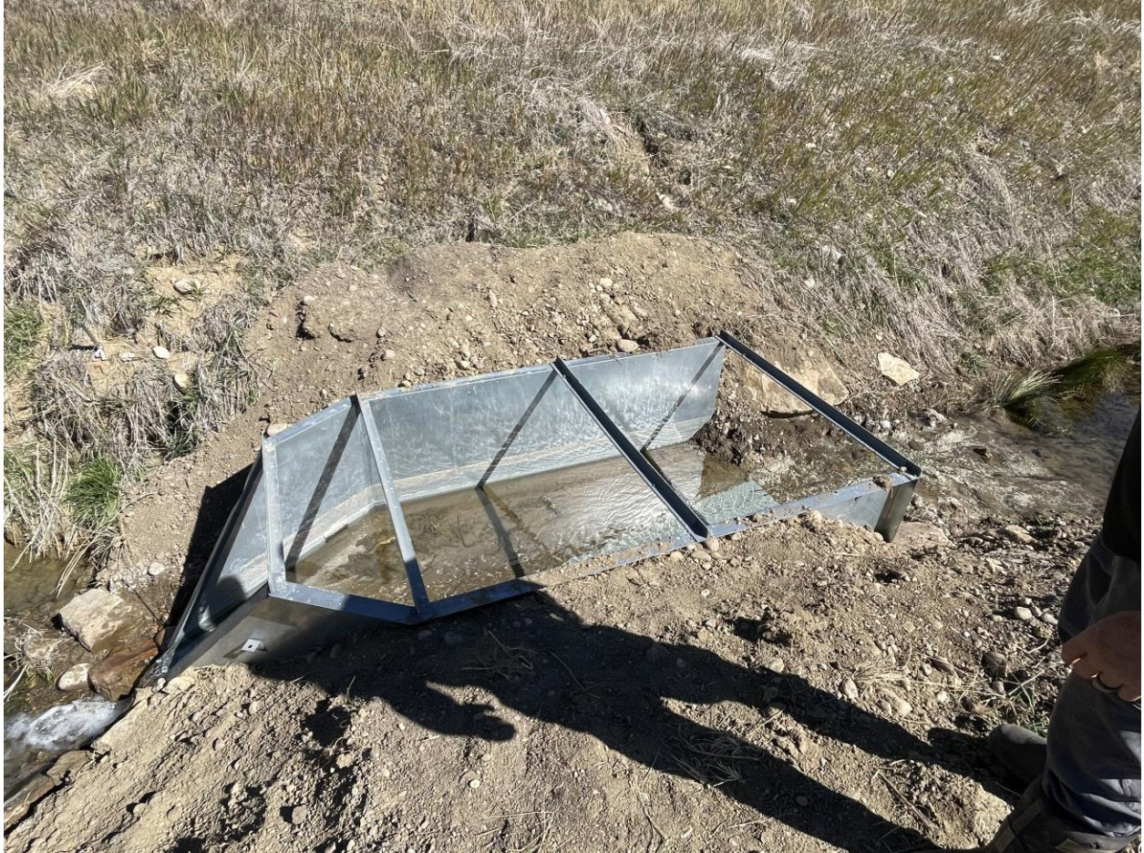
Picture 3 – New flume at Pond 2
