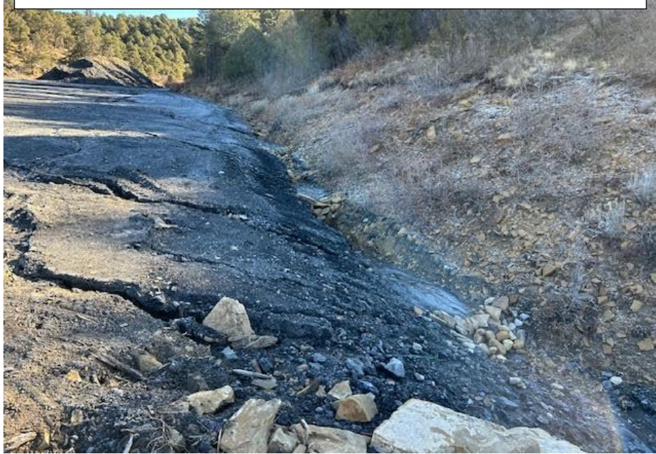
Photo 1: The upper portion of Rach 10 on top of the URDA.
