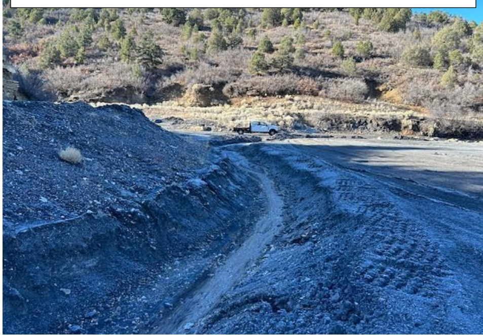
Photo 3: The portion of Reach 10 on top of the LRDA.
