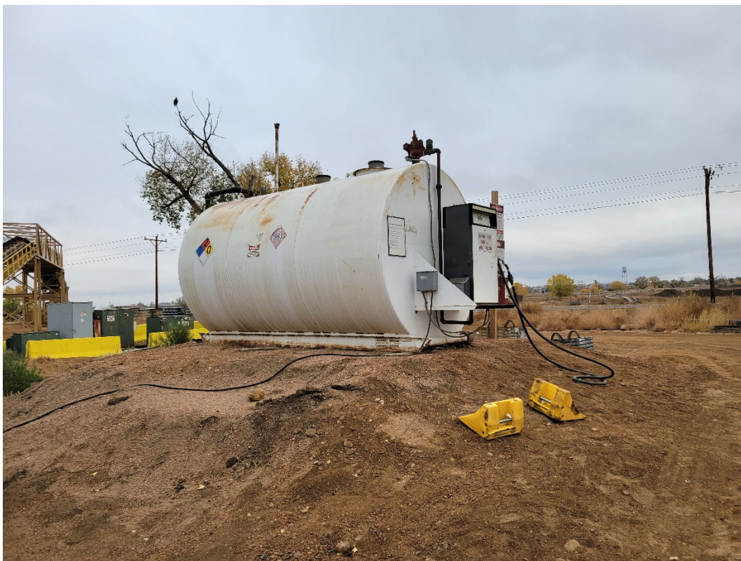
Photo 6: Double walled fuel tank adjacent to the office in the west mining area.
