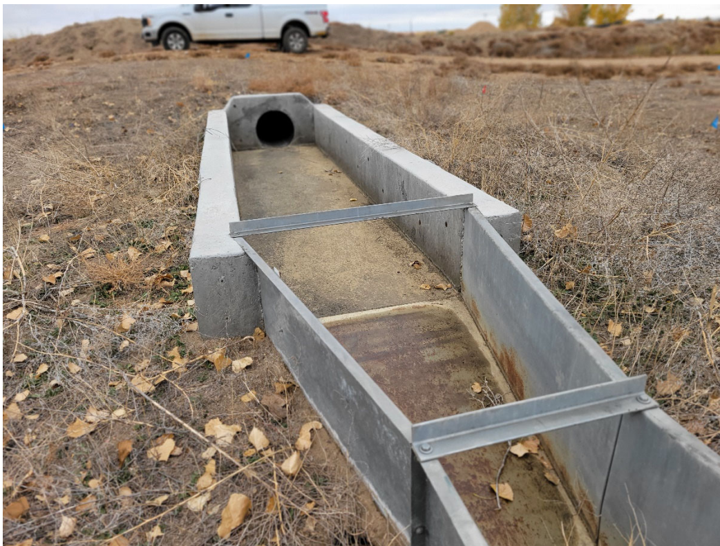
Photo 15: Discharge structure to the South Platte on the east side of the permit area.
