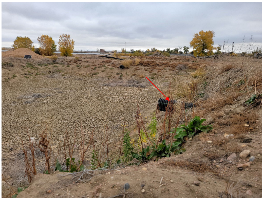
Photo 16: Settling pond east side of the permit area. Discharge pipeline indicated by arrow.
