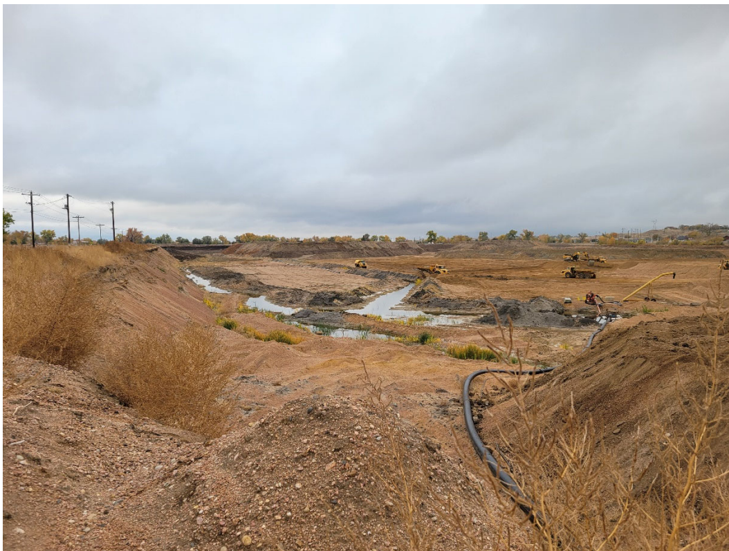
Photo 5: Groundwater trenches moving water to the sump area in the northeast corner of the west mining area.
