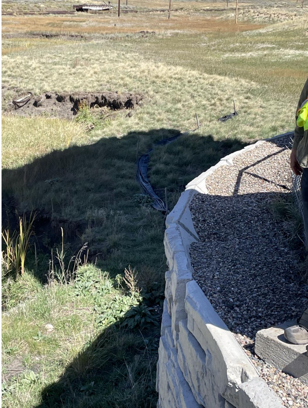
Picture 12 – Silt fence at stoker coal loadout
