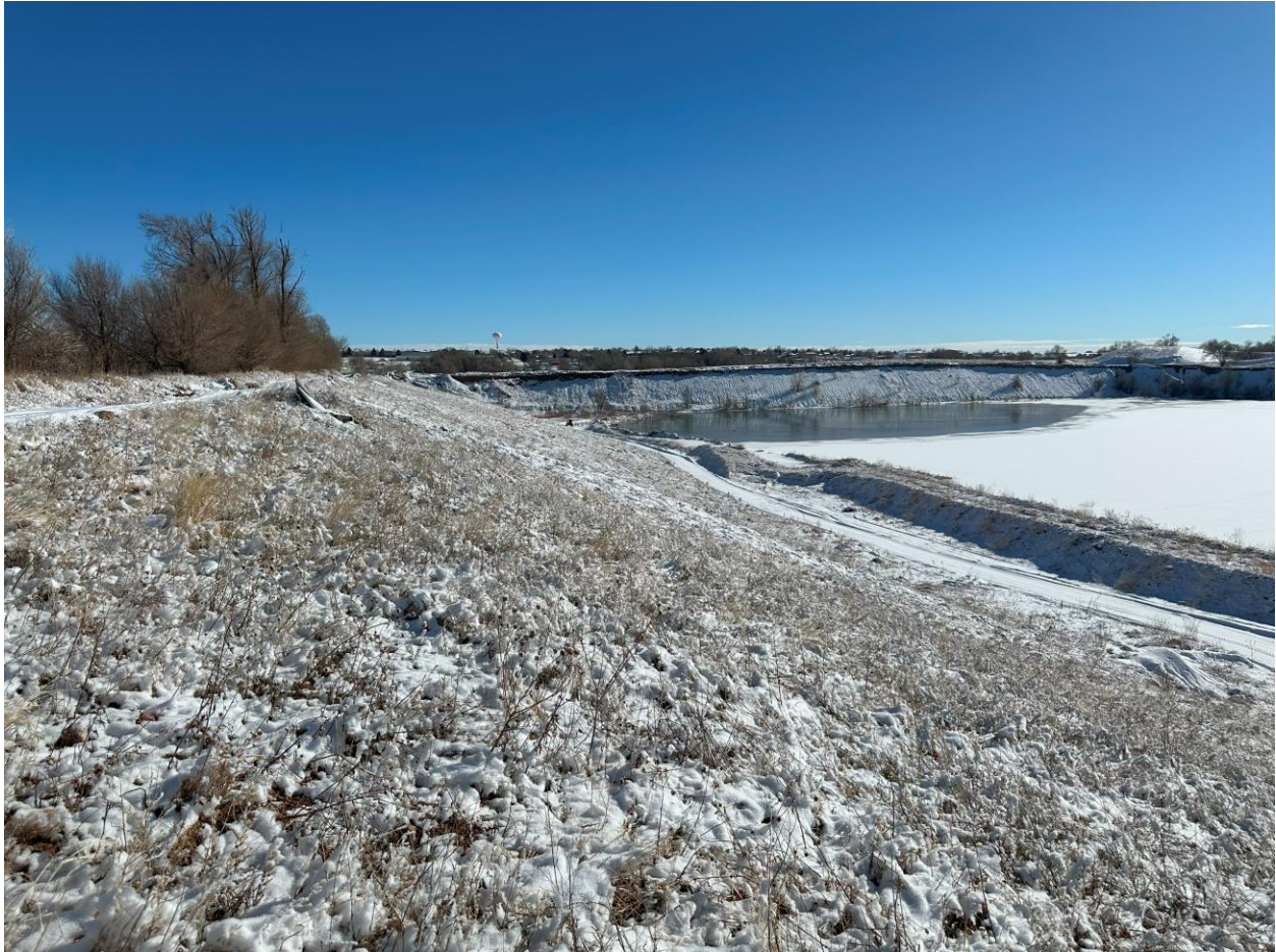
Photo 2. Buttress slope with ditch access road
