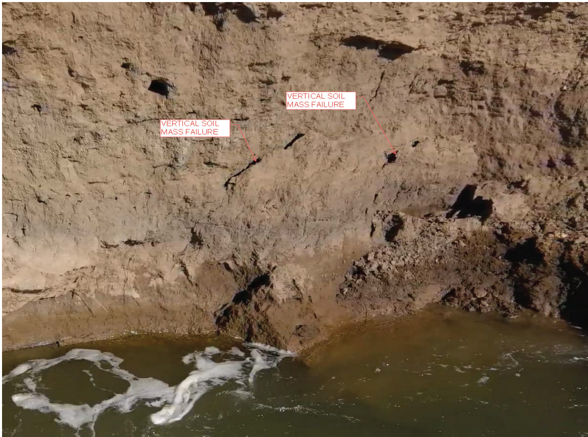
Figure 3. A Close-Up View of the Damaged Bank, Showing Where The Bank Is Failing Vertically.
