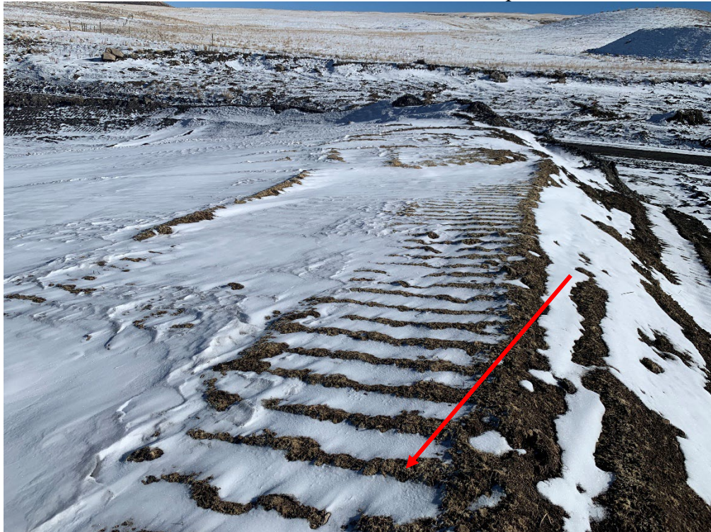
Photo 9 – Hydro seeding mulch seen in tractor tracks
