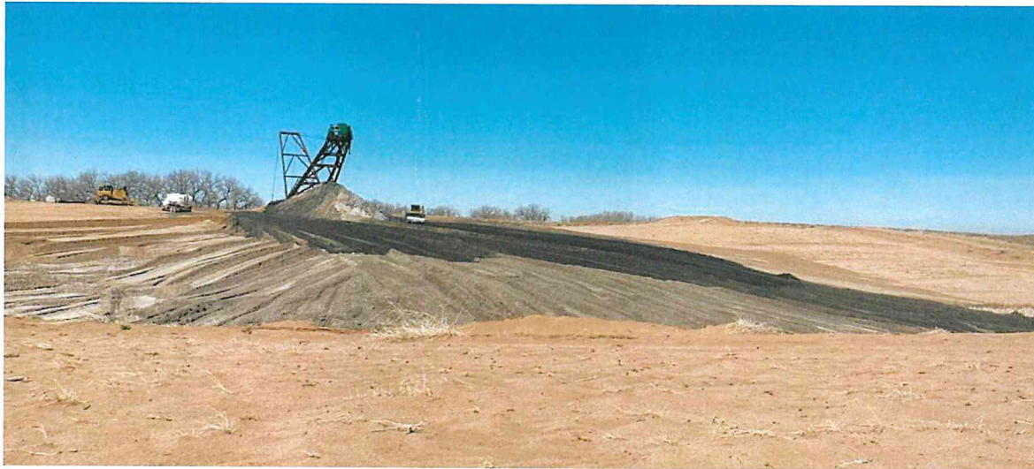
Figure 4.2: Stockpile Development Constructed from Cyclone Underflow
