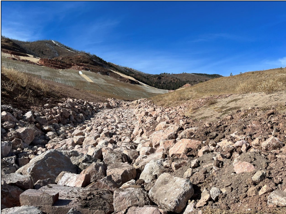
Photo 12: View northwest from inside the rip rap lined main north channel.
