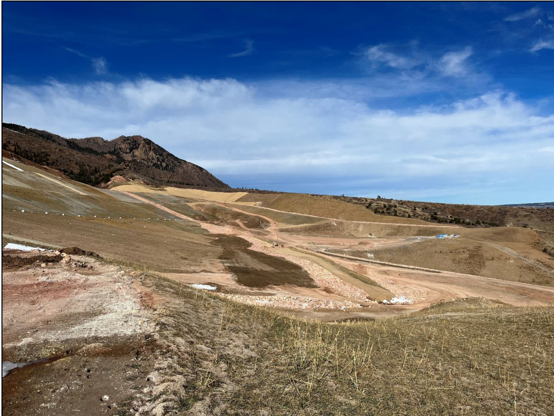
Photo 8: View north of the regraded buttress level above the Leica prism station, this addressed ponding noted in the previous inspection.
