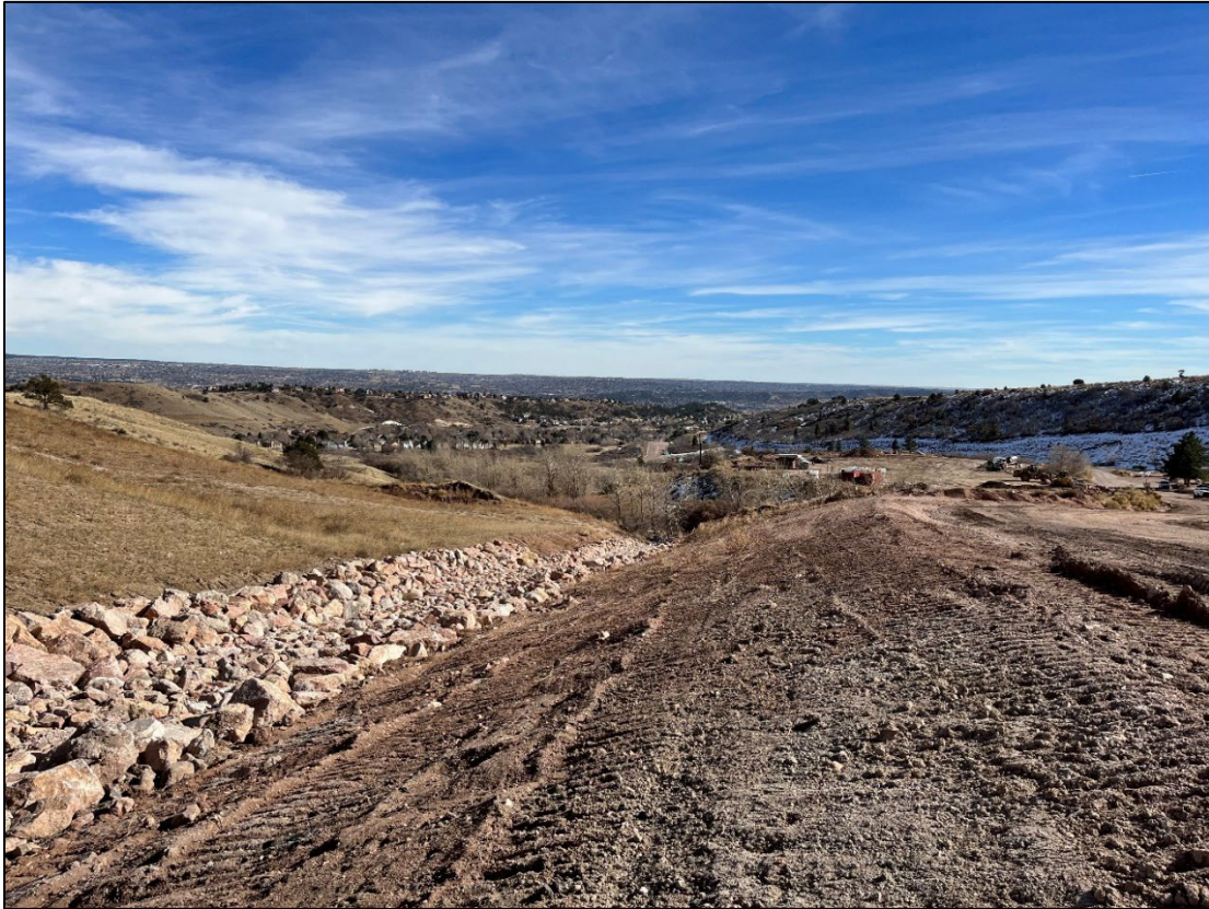
Photo 11: View east of the end of the Main North Channel and into the City of Colorado Springs Open Space area. The area to remain as a graveled lot next to the office building is also visible.
