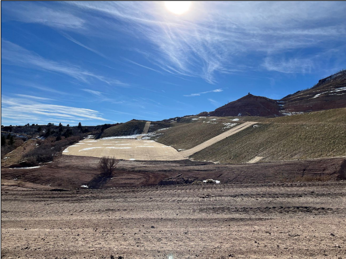
Photo 9: View south of matted slopes at the eastern edge of the buttress.
