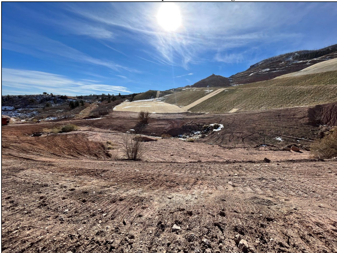
Photo 10: View south of the eastern edge of the buttress area. The culvert which connects to the slope's underdrain daylights here.
