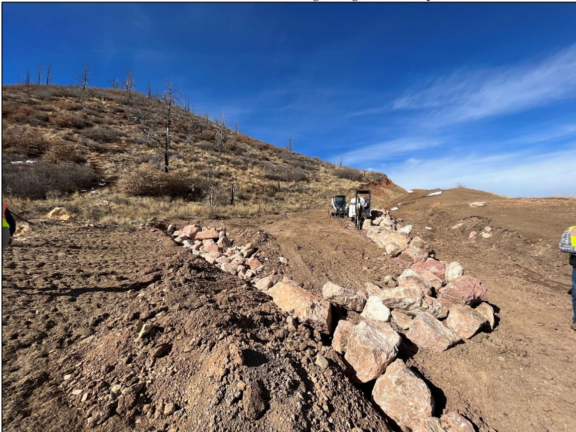
Photo 6: View west of the rock wall installed into the Upper South Channel at the request of the City and the USFS.
