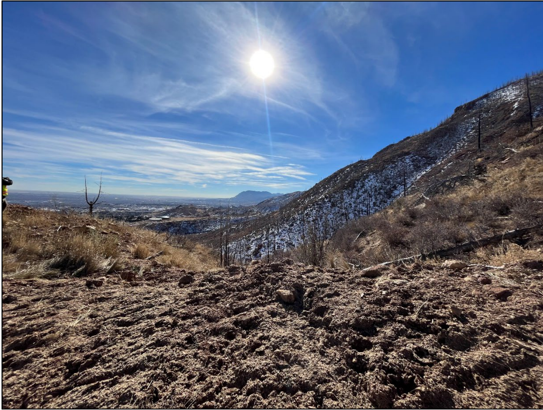
Photo 7: view south of the drainage area that has been protected from drainage by the installation of the rock wall on the Upper South Channel.
