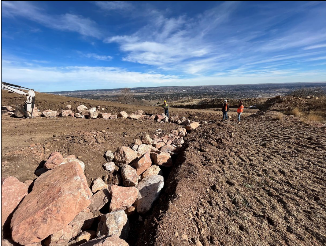
Photo 3: View of the Upper South Channel on USFS property. The rock wall is complete in this area.
