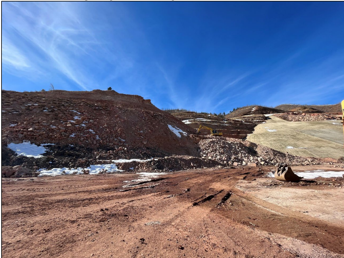
Photo 2: View of the south quarry area, rip rap is currently being removed for use on the remaining drainage channel tie-in areas.
